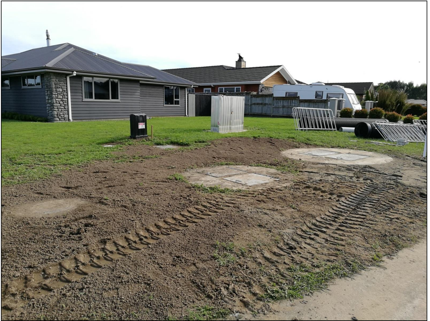
Figure 5 Okarito pumpstation - concrete apron still to be installed.
