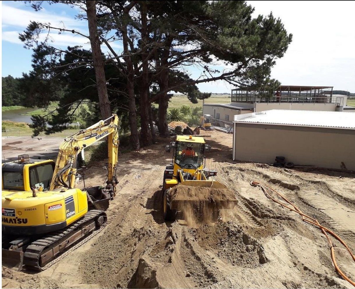
Foundation base preparation work for reservoir construction
