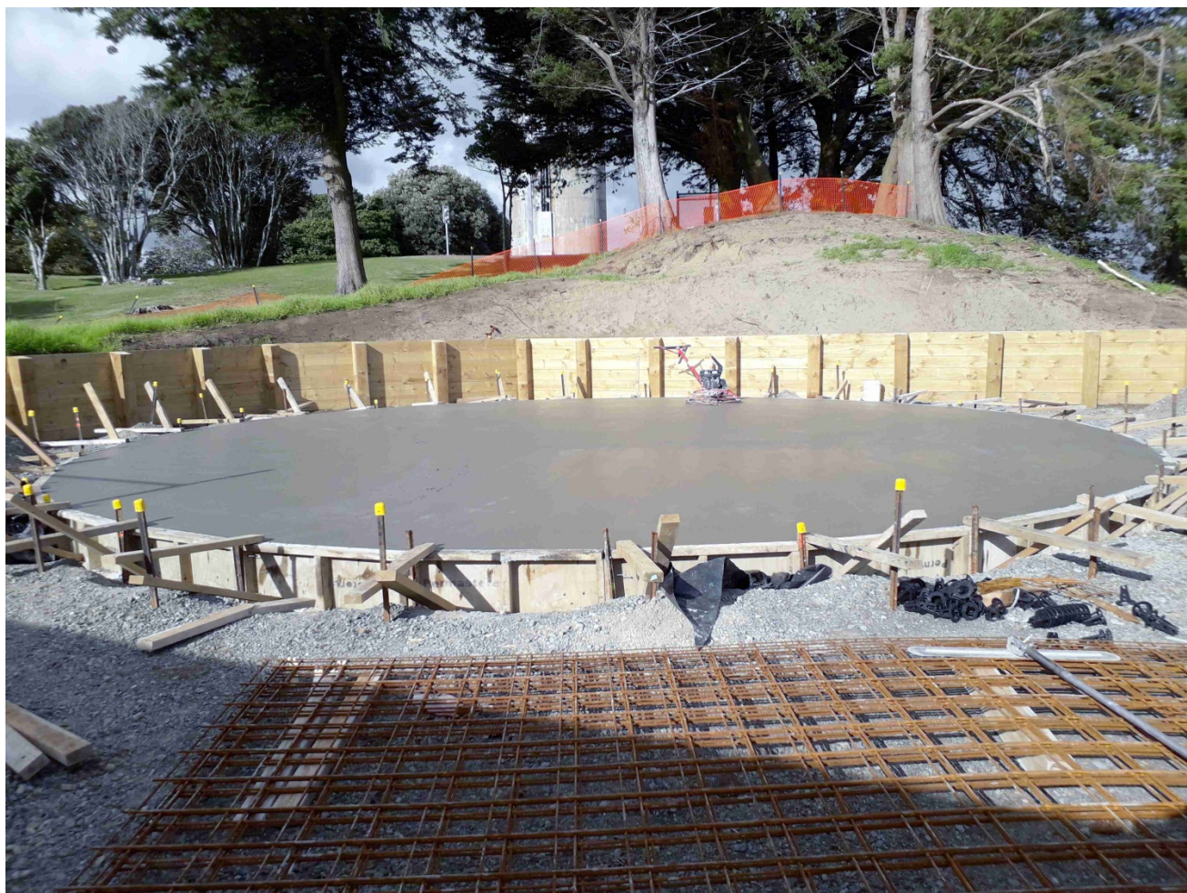
Foundation base for reservoir construction
