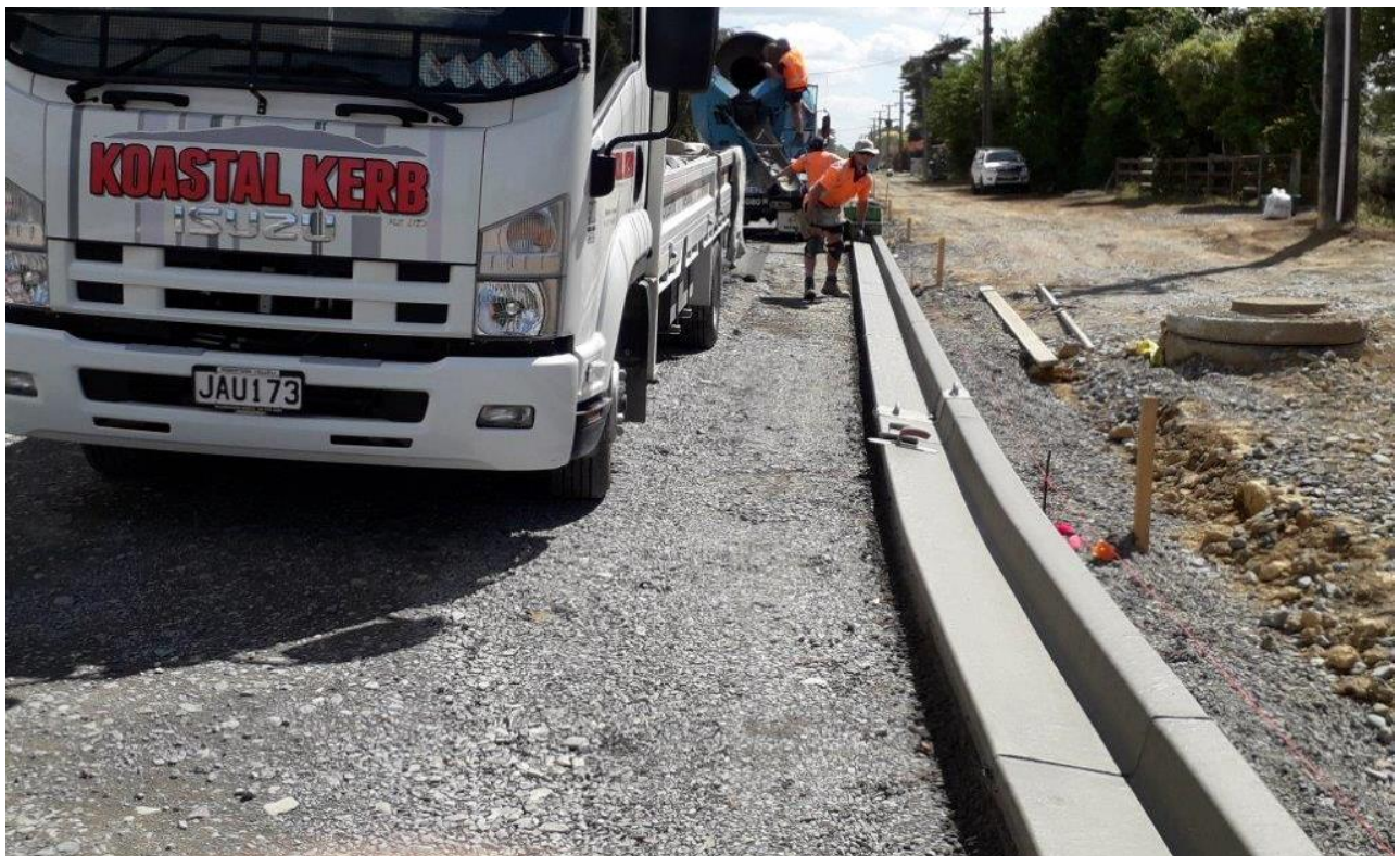
New kerbs being installed (December 2017)
