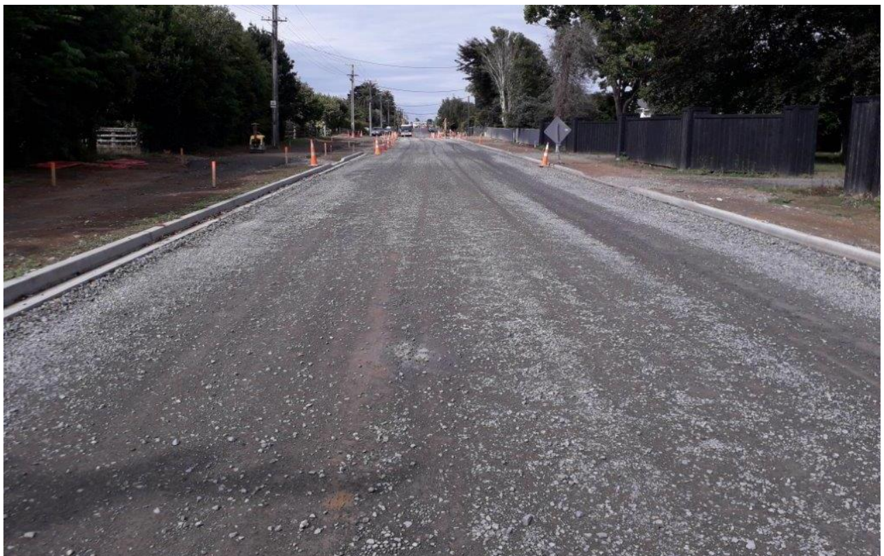
New kerbs installed (December 2017)
