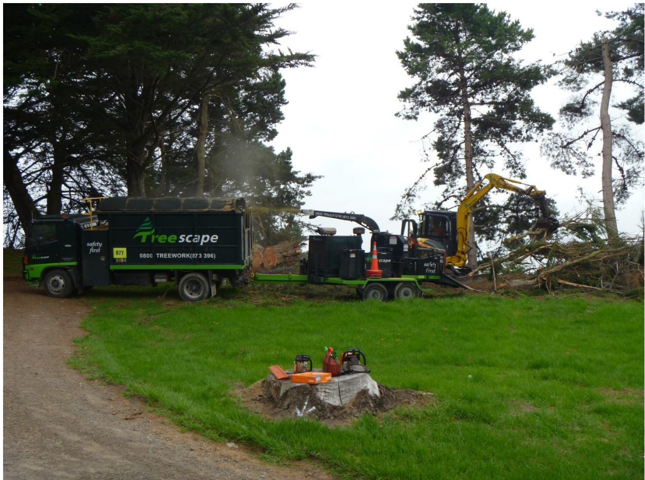
Tree removal in preparation for reservoir construction
