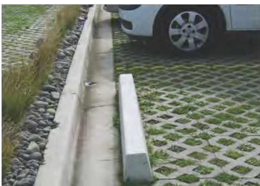
Permeable paving used where possible and stormwater managed on site
