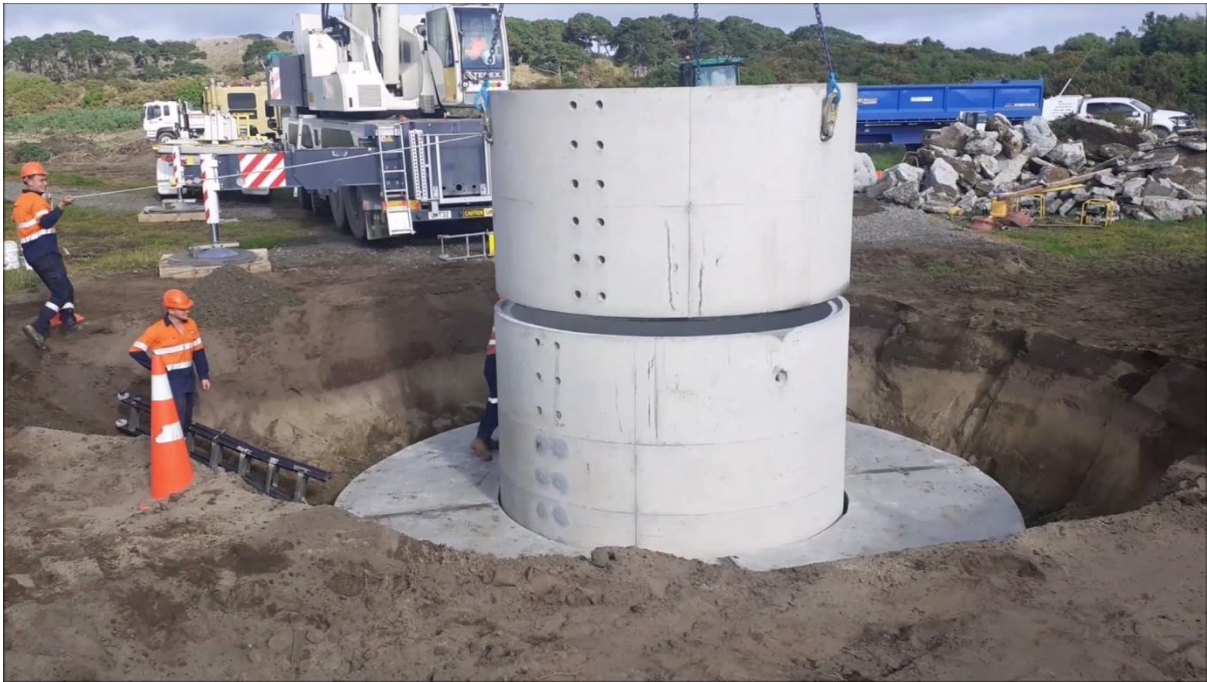
Adding the top half of the new wet well
