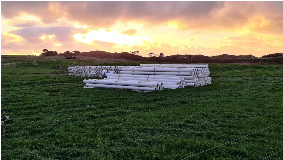
Irrigation mains pipes delivered to site ready for installation
