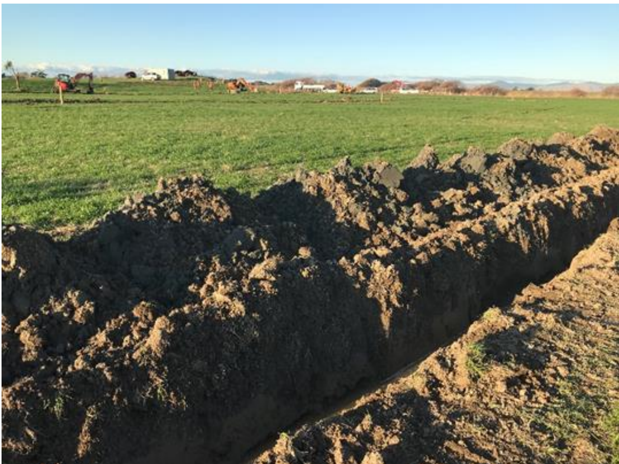
Trenching to install irrigation pipelines
