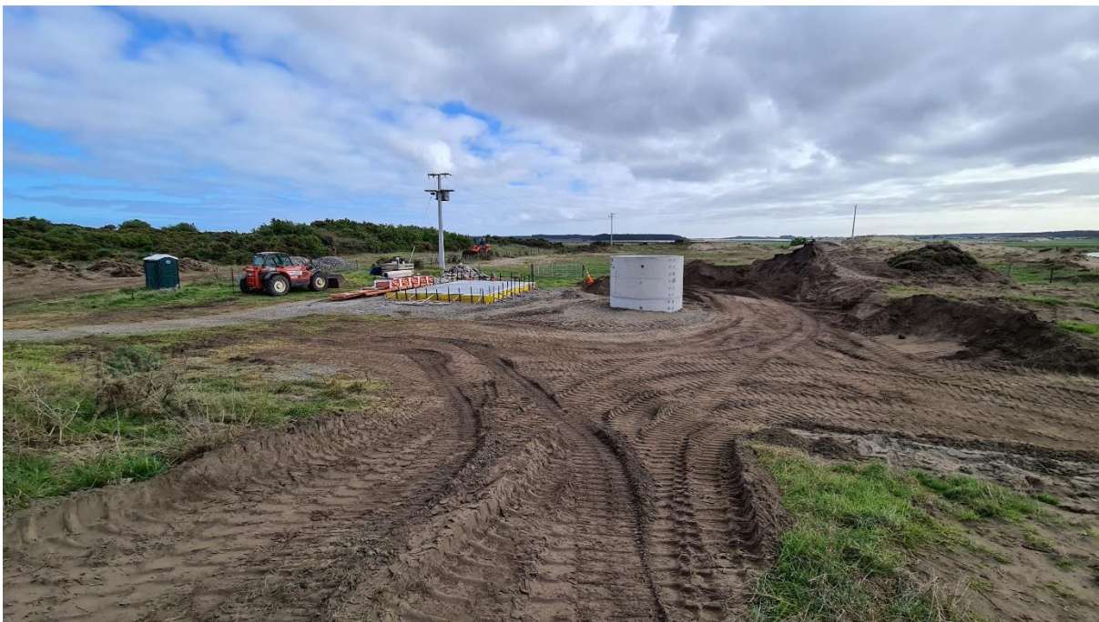
Wet well and foundation for pump shed
