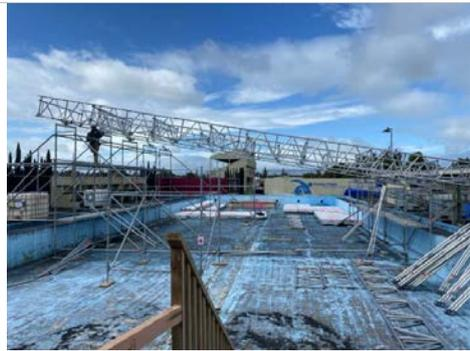
*Construction of the temporary painting tent that will be used to paint materials before they are installed.*
