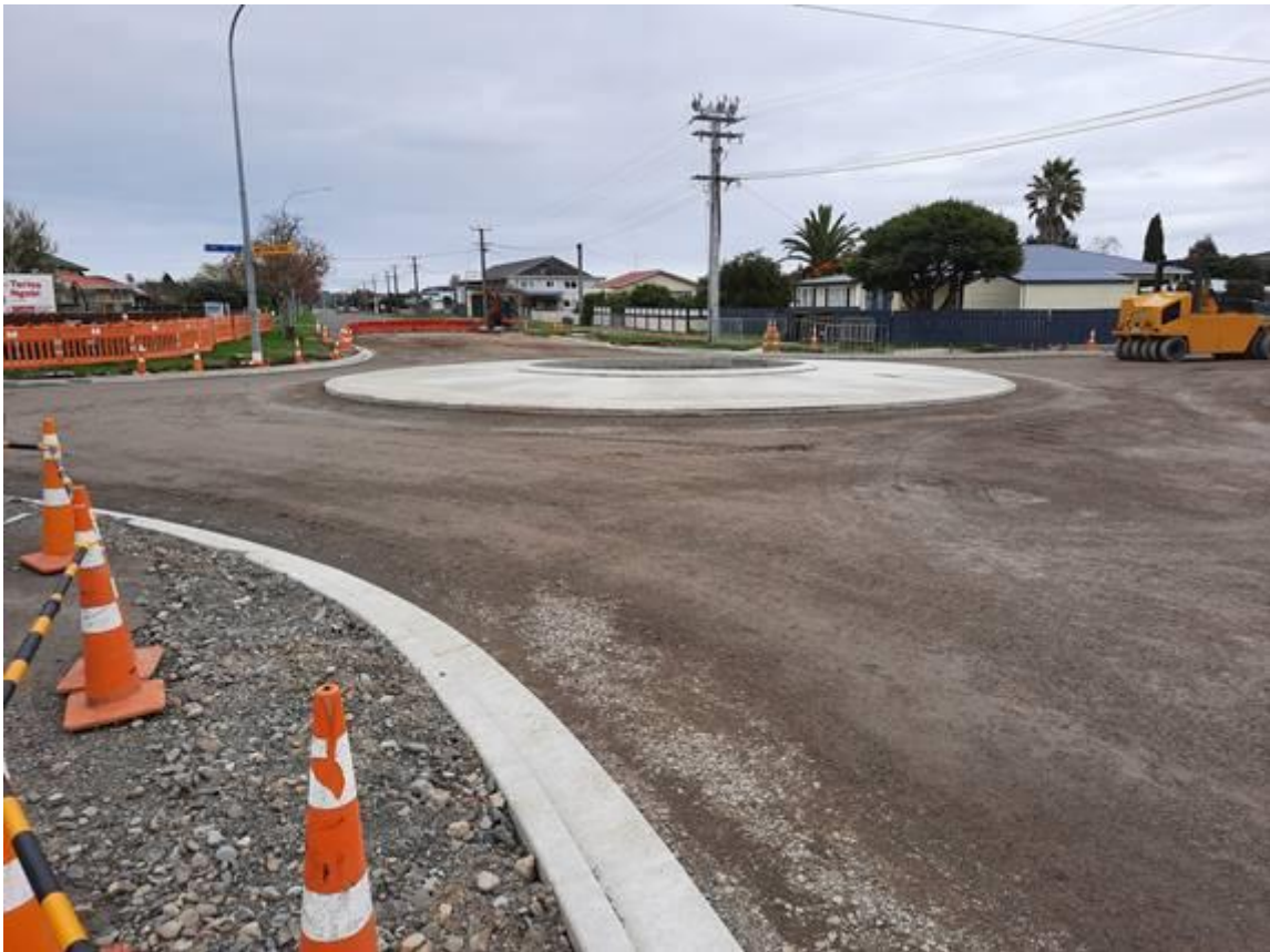
Queen Street / Tiro Tiro Road Roundabout Project well under construction.
