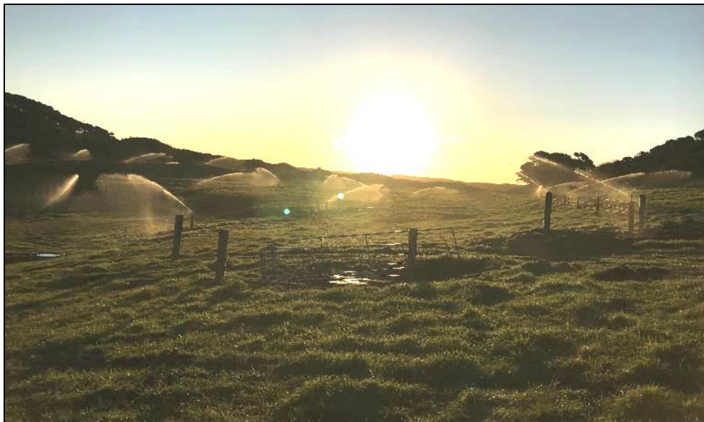
Pre-commissioning flushing and pressure testing of irrigation sprinklers.
