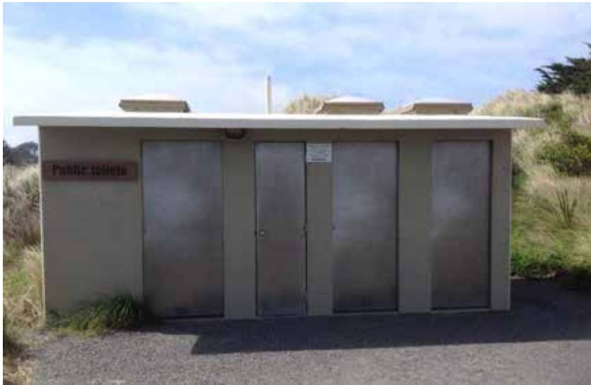
Image 13 Public toilets in the car park at Waitarere Beach
