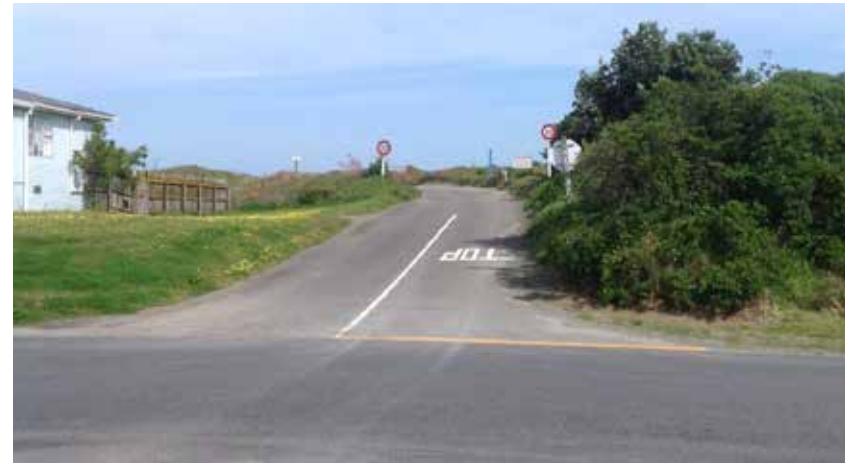
Image 7 Alternative vehicle access to Waitarere Beach from Windsor Street
