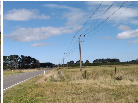
Fenced off berm Foxton-Shannon road
