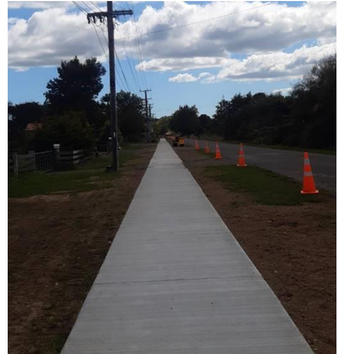
New footpath completed.
