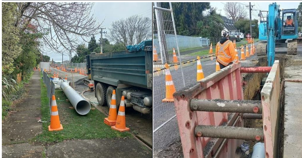
Kings Drive Sewer 475mm upgrade
