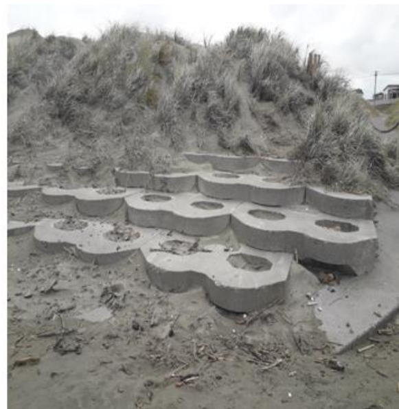
Photos of localised erosion resulting in subsidence and damage of seawall
