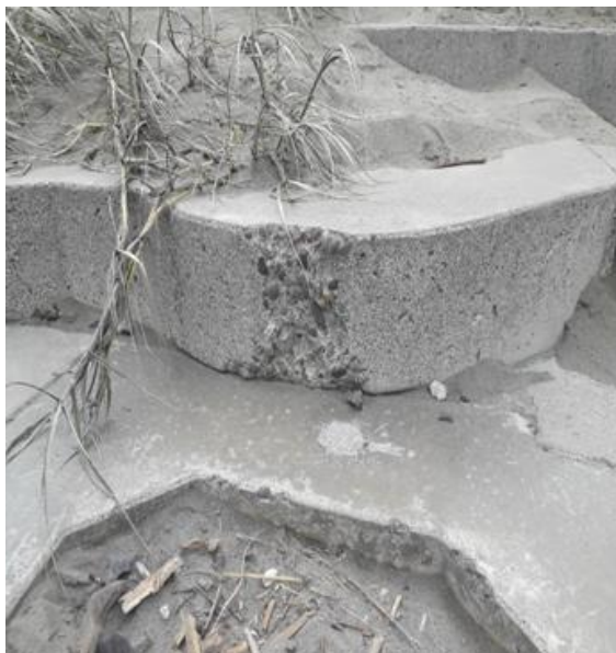
Photos of localised erosion resulting in subsidence and damage of seawall
