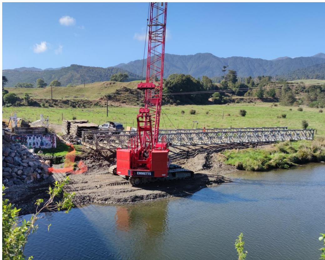
Old bridge down for disassembling
