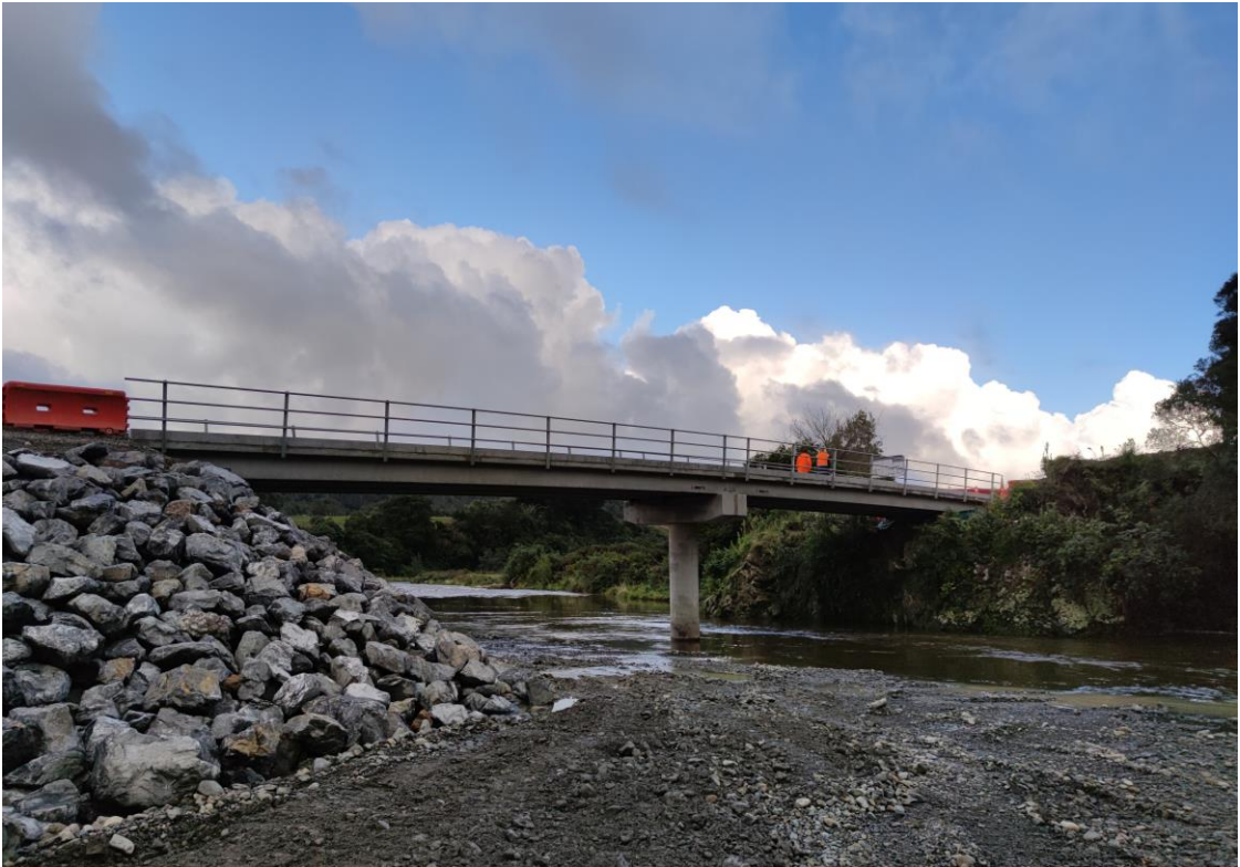
New bridge with completed riprap rock protection on the eastern abutment
