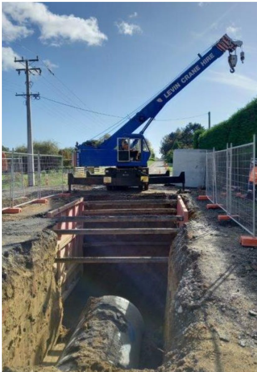
New 1500mm diameter stormwater pipe installation
