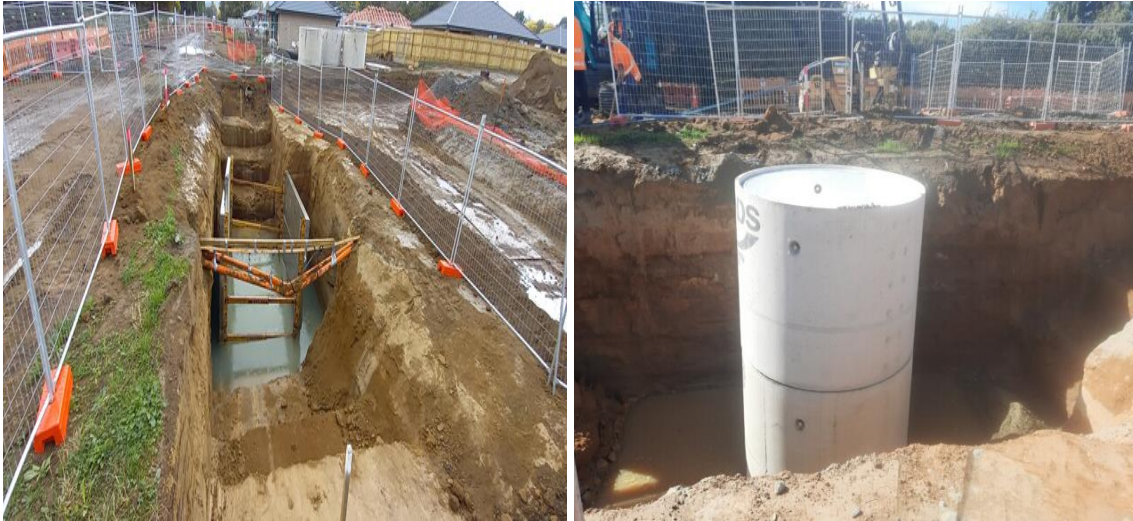
Roslyn Road new wastewater pump station, before (left) and after (right)
