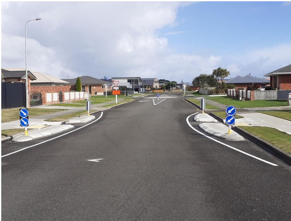
Traffic island build-outs and mountable roundabout on Andrews St
