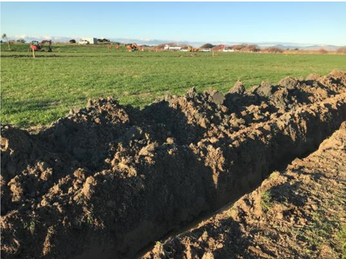
Trenching to install irrigation pipelines
