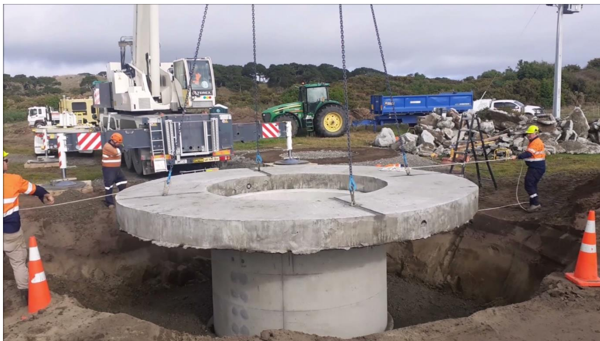
Installing ballast ring around bottom half of new wet well
