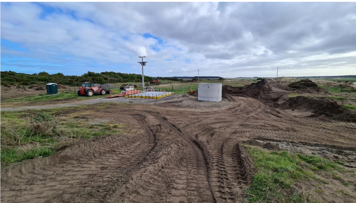
Wet well and foundation for pump shed
