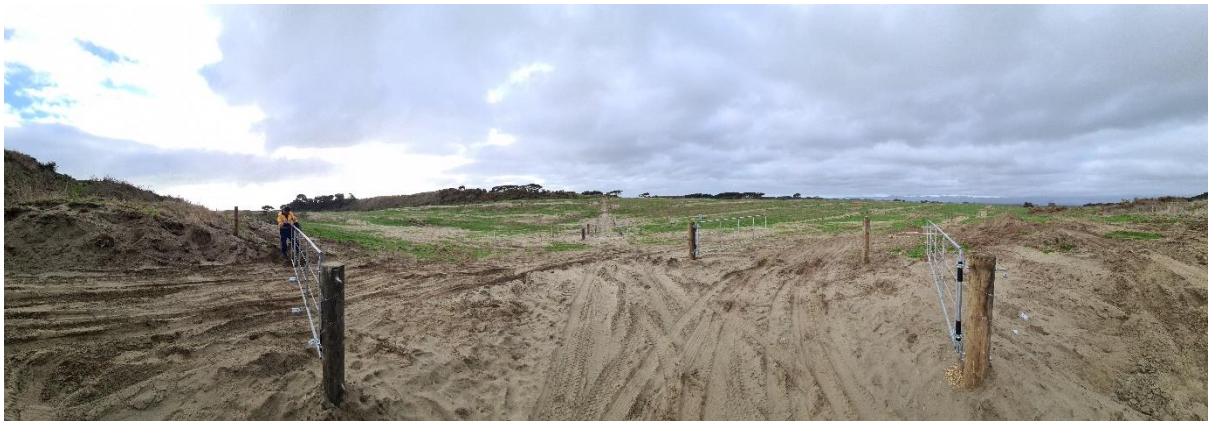
New stock route, paddock gates, and fencelines ready for irrigation to be installed
