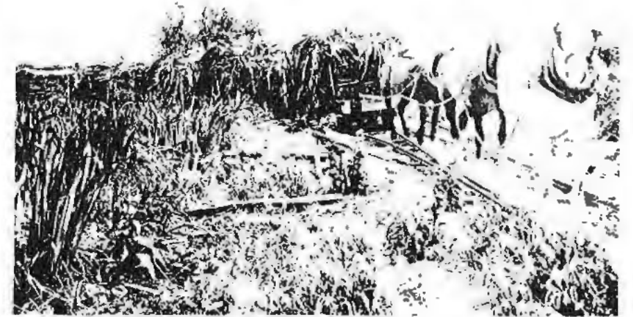
(15) Right: When the locomotive proved too heavy for the track in the swamp, horses were used to pull the flax-laden wagons or trams to the mill. Two of these powerful animals, half light and half draught, hauled five trams and three horses were needed to pull a train of 9 trams. Each tram when fully loaded weighed over a ton. Over 70 horses were used to carry out the various tasks at the mill and in the swamp. In 1920 the horses were replaced with motor trucks. The "trammies" drove the horses and laid the rails into the blocks of flax. Over 11 chains of tramlines were pulled up and relaid every day. Photo: Palmerston North Public Library.
