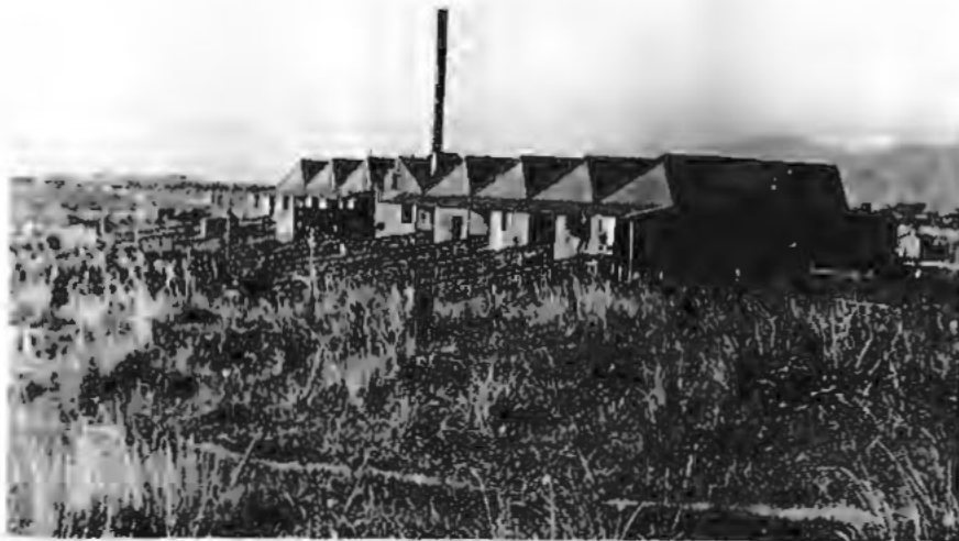
(18) Left: A view of the stripping shed taken in the 1920s. Note the differences between this photo and the earlier one. A tall chimney stack has been added and seven sets of rails run right into the building to feed the stripping machines. Photo: Palmerston North Public Library.
