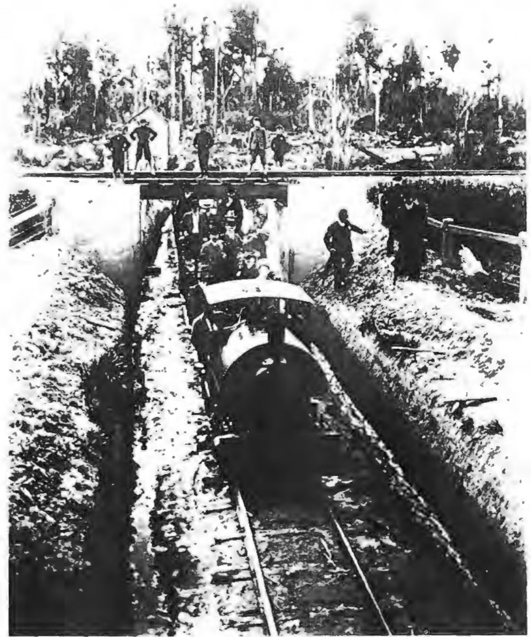
(4) The mill's five ton "Bagnall" locomotive carrying guests and members of the press on the day of the official opening. They are returning from a tour of the Makerua flax swamp. The engine is passing beneath the railway line owned by the Wellington-Manawatu Railway Company which passed the mill. The mill owners paid the railway company the sum of 1 pound for many years for the right to pass beneath the line. Photo: Palmerston North Public Library.
