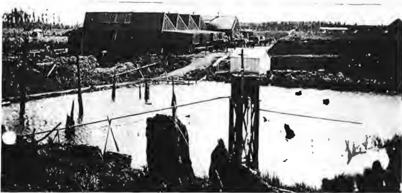
(17) Above: A rear view of the stripping shed in the early days with the 750,000 gallon reservoir in the foreground. The water was used to wash the flax fibre during the stripping process. Photo: J. McNeile.
