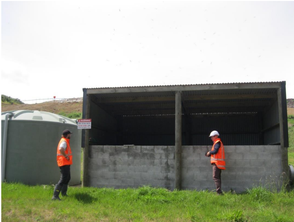
Figure 7: Biofilter structure at the toe of closed landfill Area A3.
