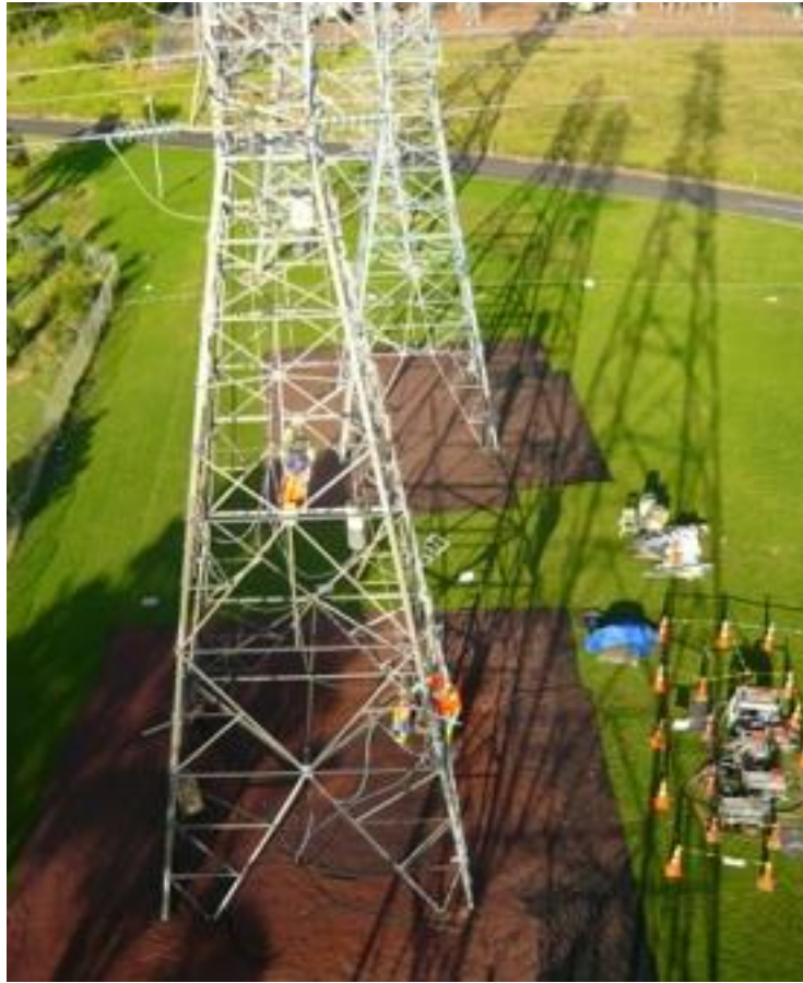
Photo 8: Use of geotextile matting
