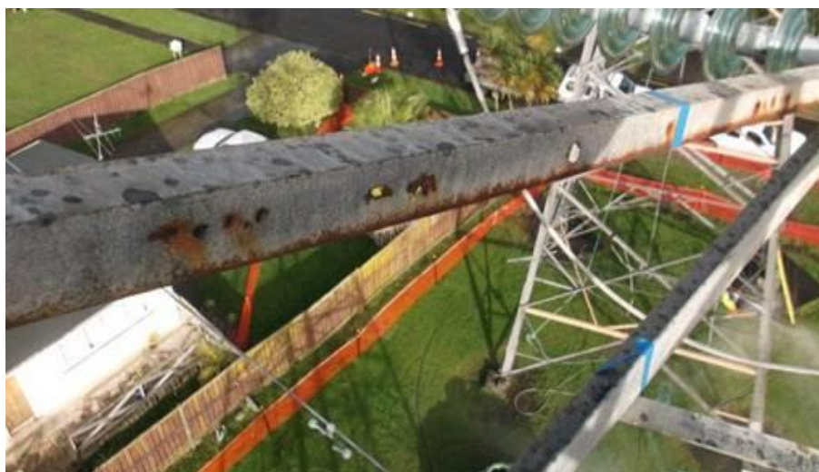
Photo 2: Tower corrosion
