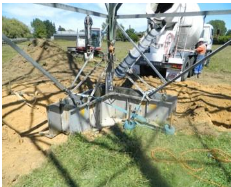
Photo 1: Typical grillage foundation strengthening
