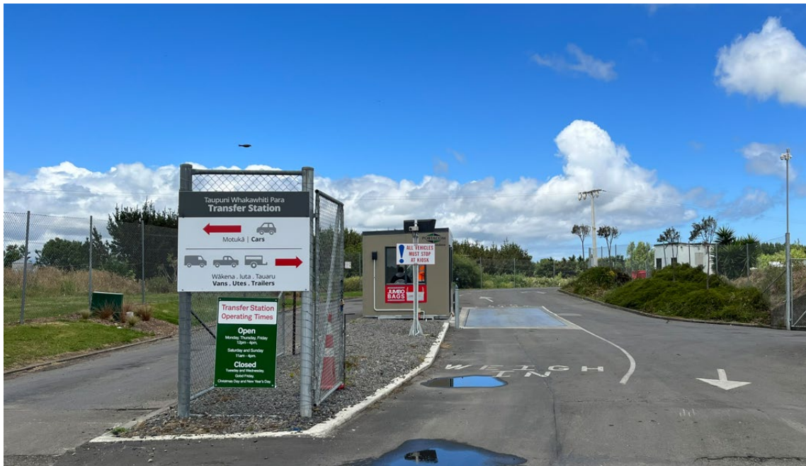
Foxton Transfer station entrance
