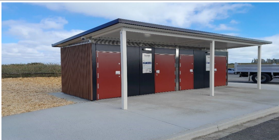
New Waitārere Beach toilet block
