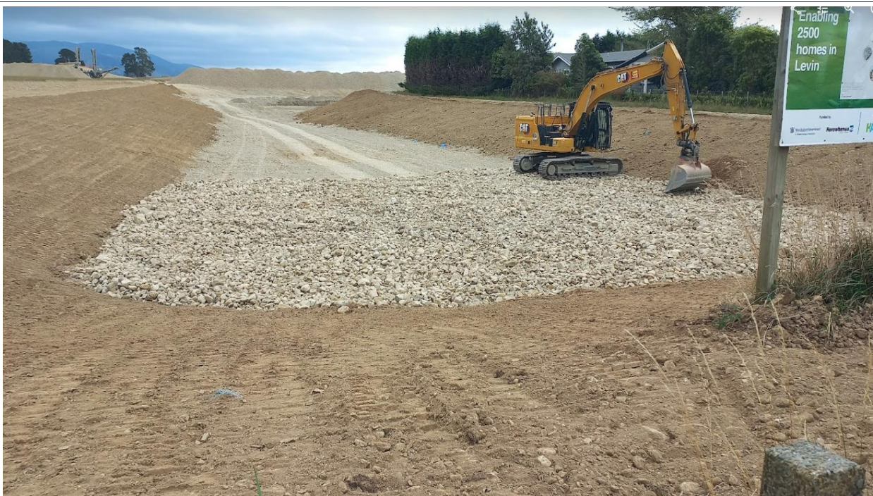
Bulk earthworks for the first stage of Tara-ika
