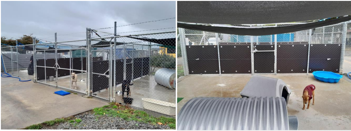
New separation panels added to the dog exercise areas at the pound
