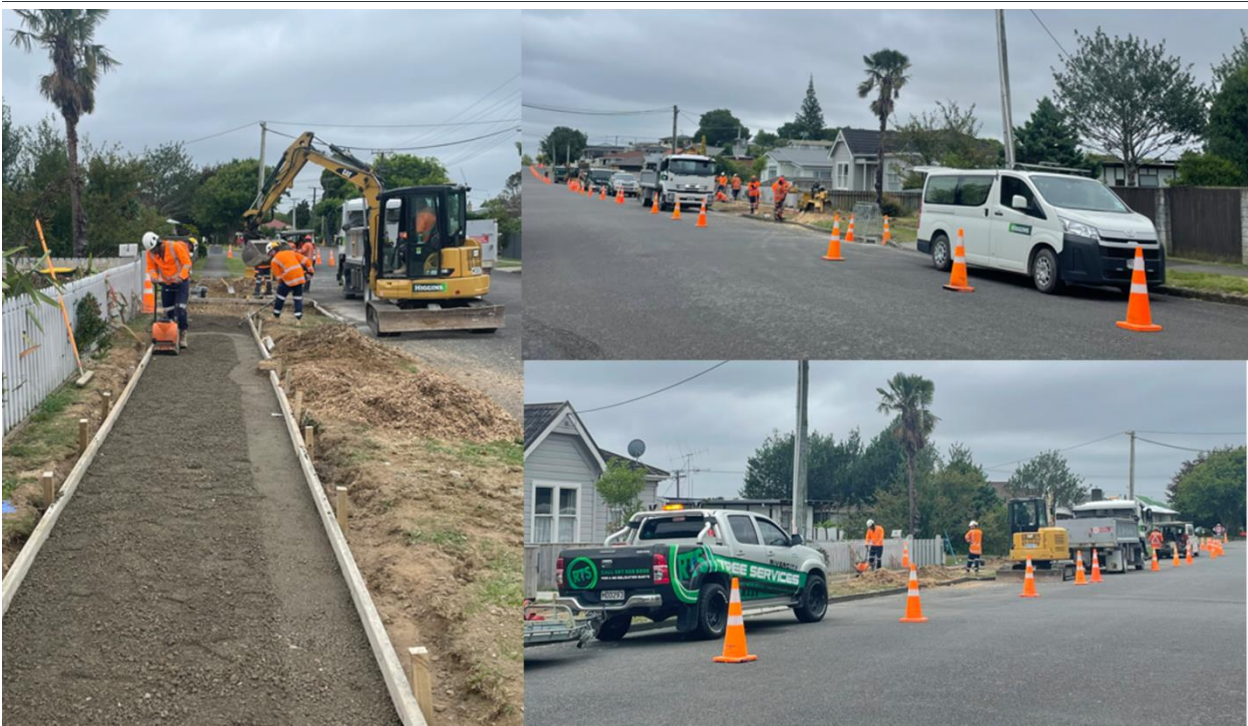
Winchester Street Footpath Renewal
