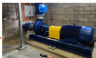
The refurbished pump and motor after installation
