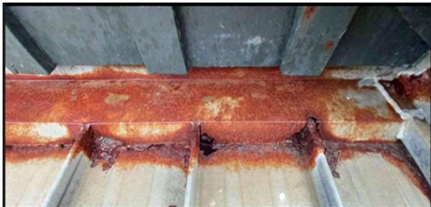
Holben Pavilion Roof
