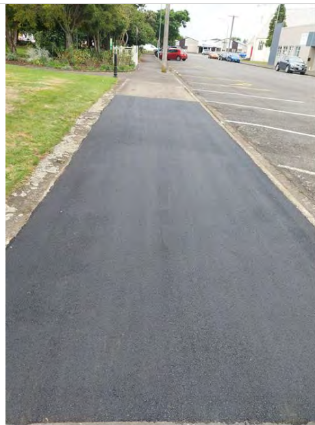
Asphalt footpath maintenance completed in Kent Street outside Thompson House.
