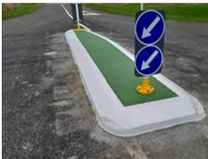
Vance street Island completed, with a lovely paint job.
