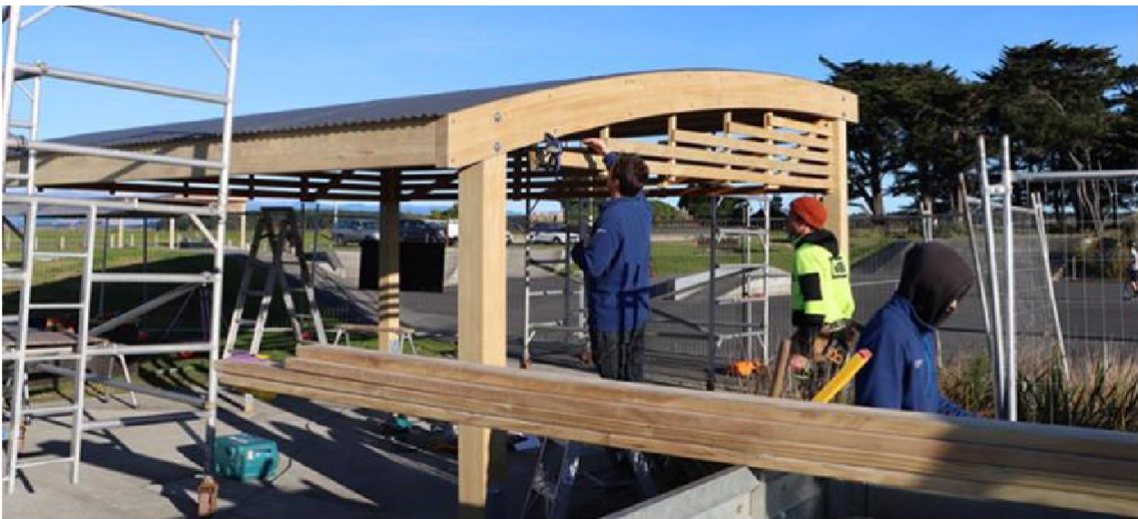
Finishing touches to the most recent BBQ shelter Holben Reserve
