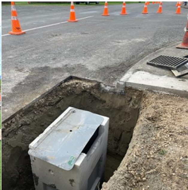
Part of the Ramona Ave / Forest Road drainage improvements
