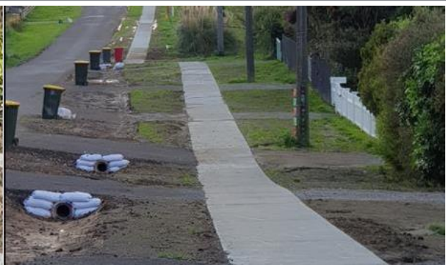
Roadside Drainage Improvements
