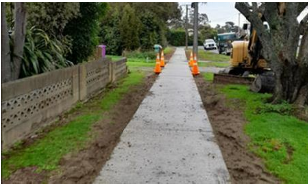
Julyan Street Shannon - footpath renewal
