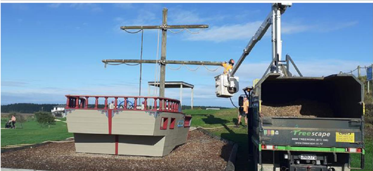
Installation of new rope on Jones playground Ship (Flagstaff reserve)
