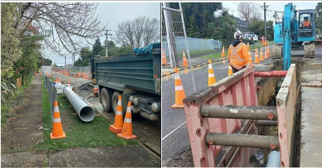
Kings Drive Sewer 475mm upgrade
