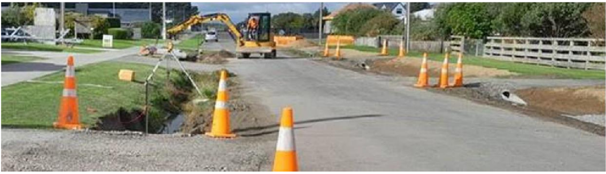
Cousins Ave West, Foxton Beach Drainage Improvements
