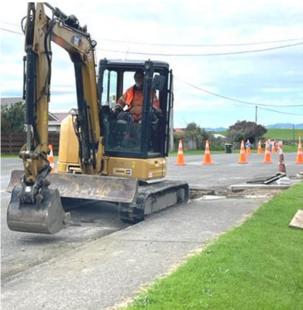
1 Waitare Beach Road. Catchpit installation
