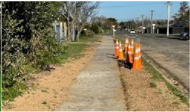
Rata Street, Tokomaru - new footpaths
