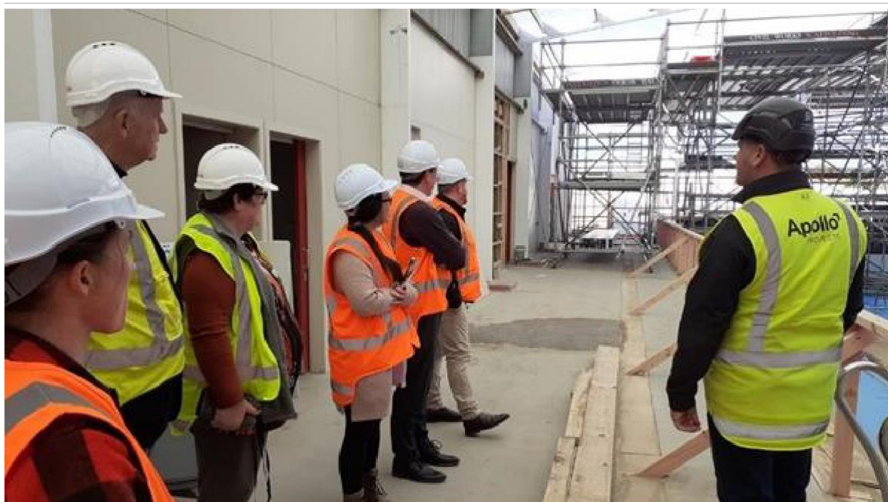
Photo above; Elected Members, Executive leaders and Te Awahou Foxton Community Board members listening to the Project Manager at Foxton Pool.
