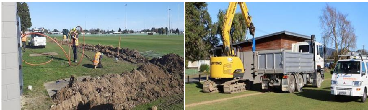
Cable trenching floodlights at Playford Park and post auger.
