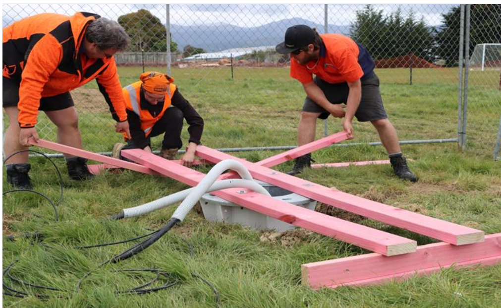
Image 6: Installation of Floodlight Footings Donnelly Park
