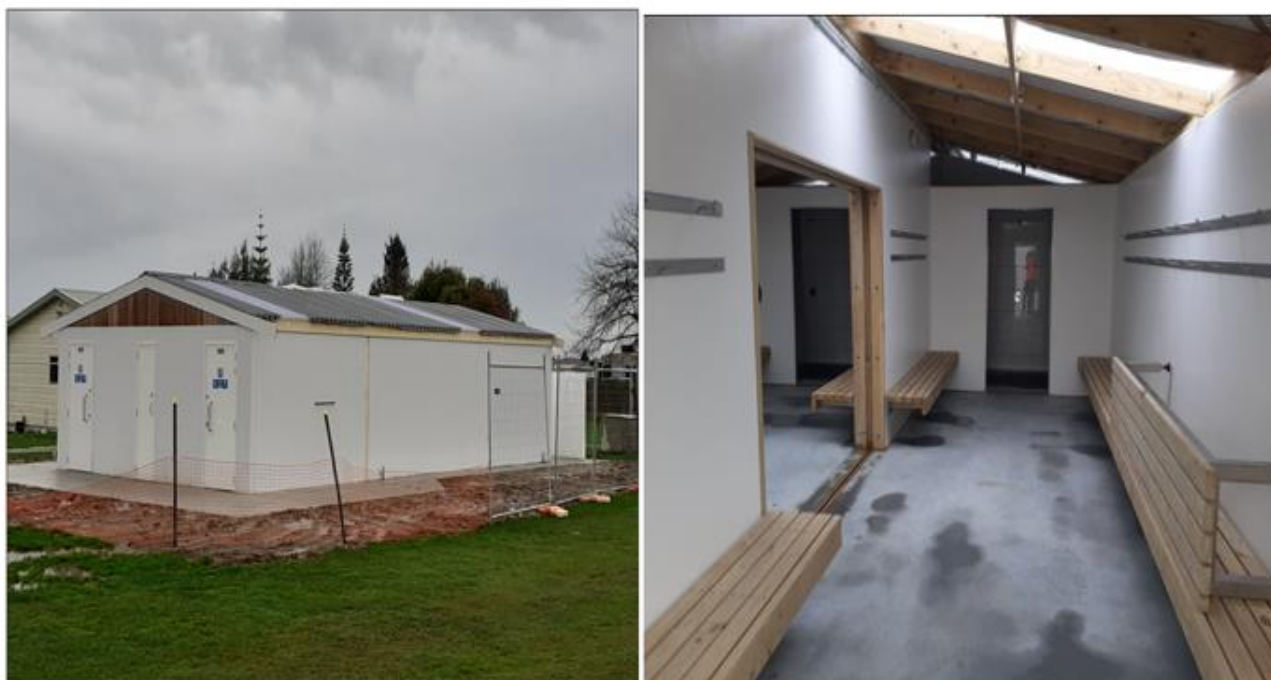
Image 1: Completed Ablution Block Playford Park
