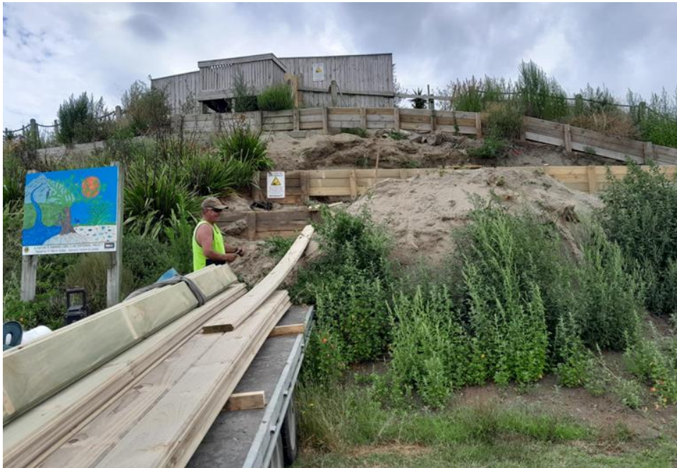
Flagstaff Reserve Remediation Works
