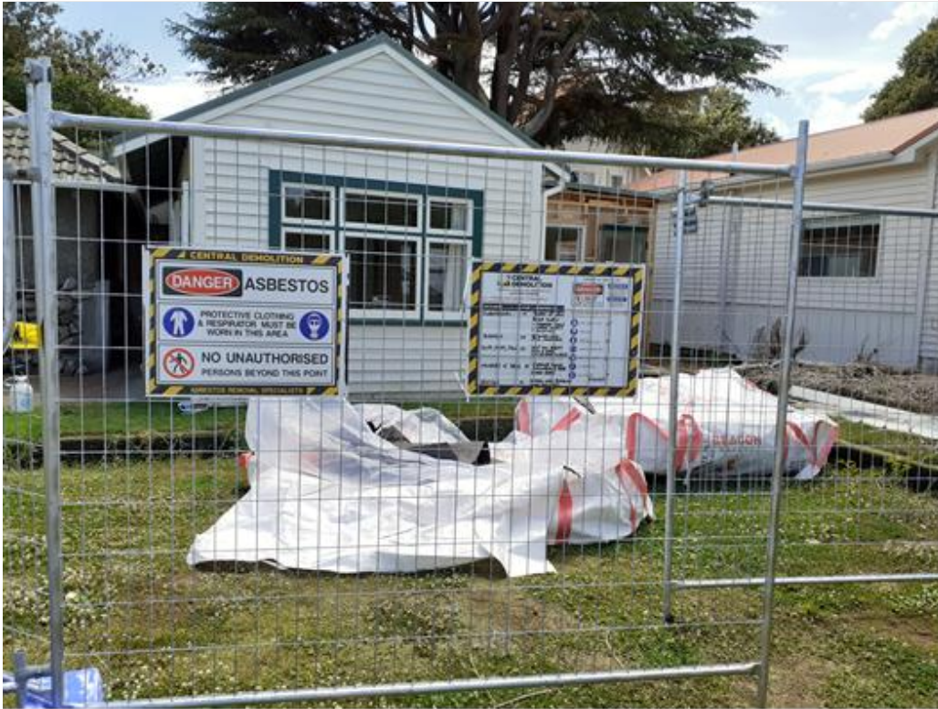
Site signage and asbestos bags at front of site (above)
