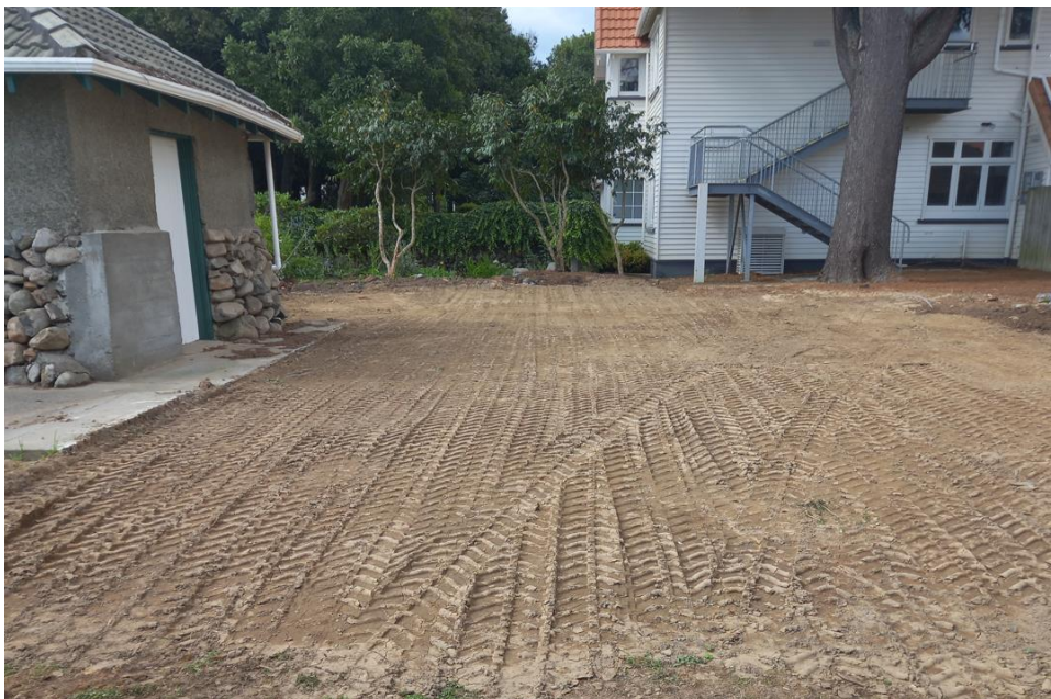
Site of ex Bowling Club reinstated with topsoil
