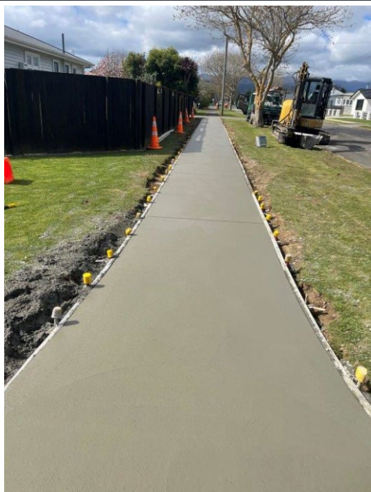
Dudley Street Footpath Renewal
