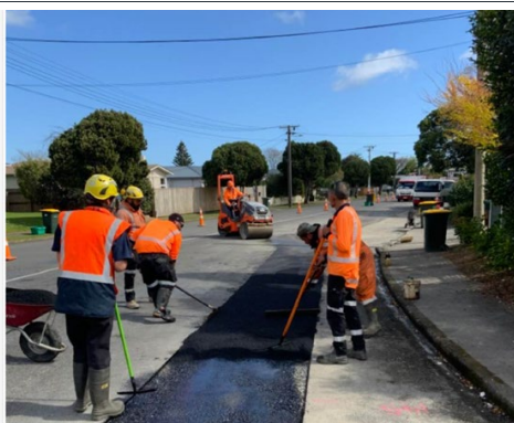
Renewal of wastewater pipe
