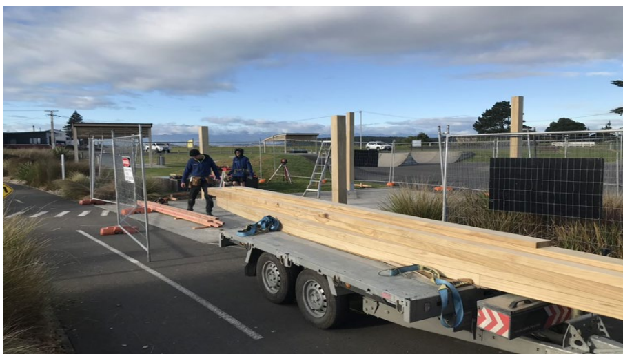
New Shelter being installed at Holben Reserve
