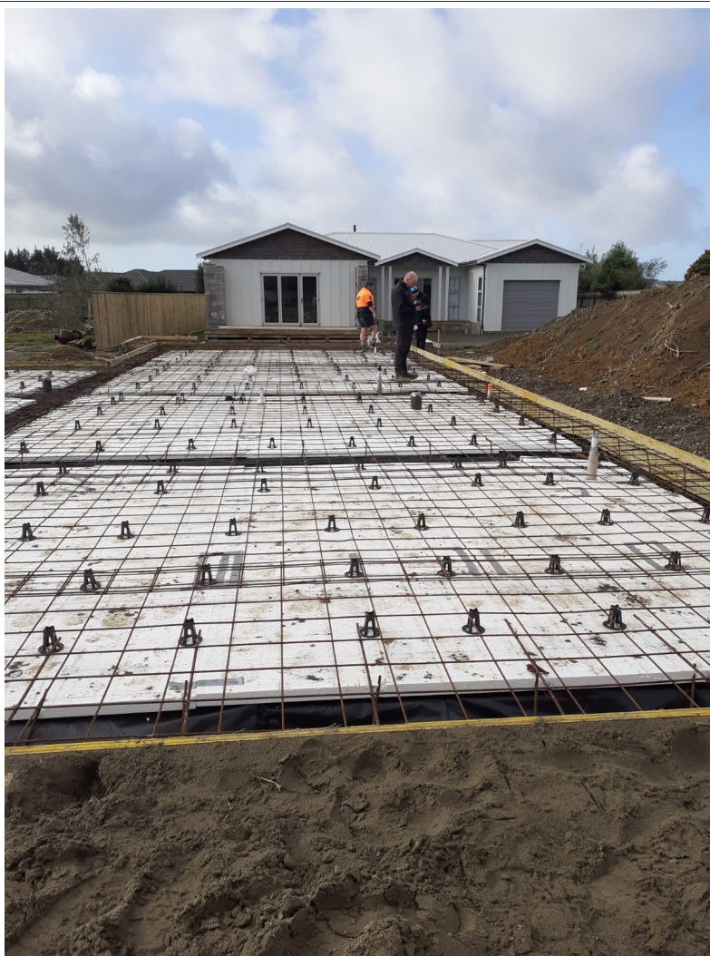
Building Advisory Officer inspecting building site – pre-concrete pour.
