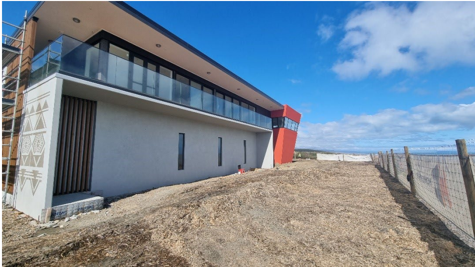
Waitārere Surf Life Club construction
