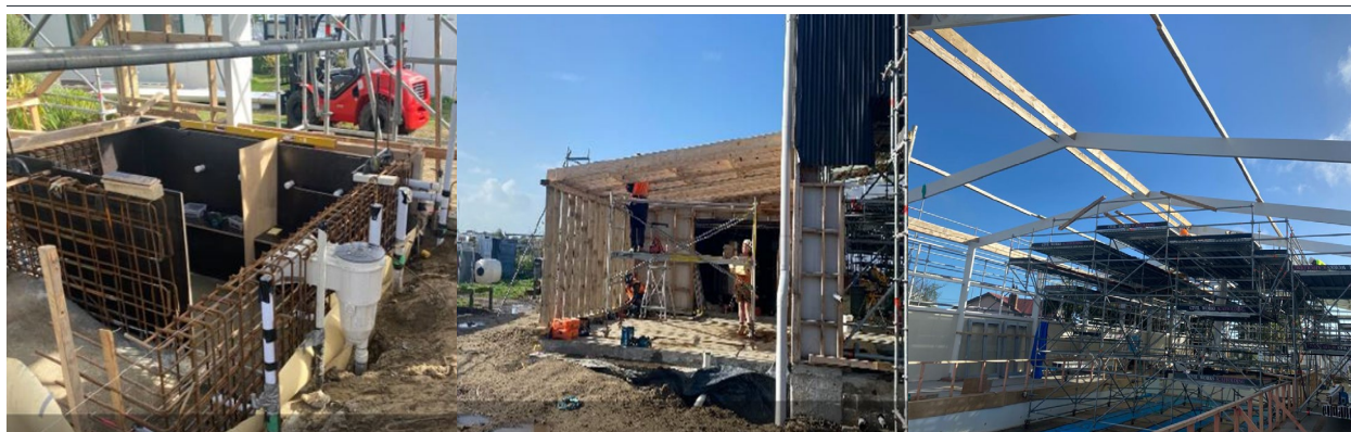
Construction of the new spa pool
