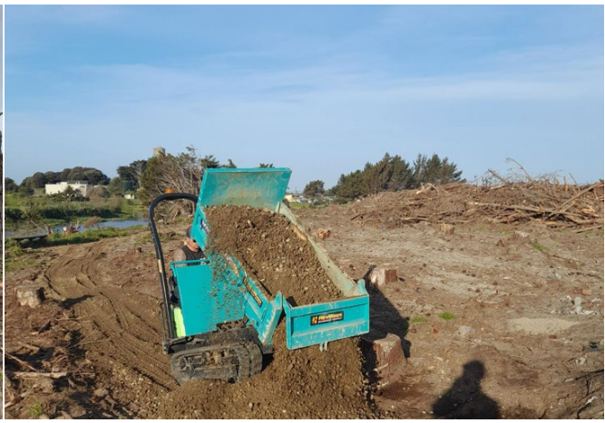
Application of base course to Piriharakeke Walkway
