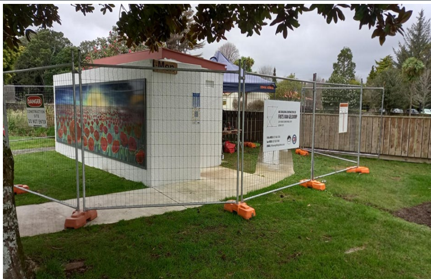
Works at Levin public gardens toilets
