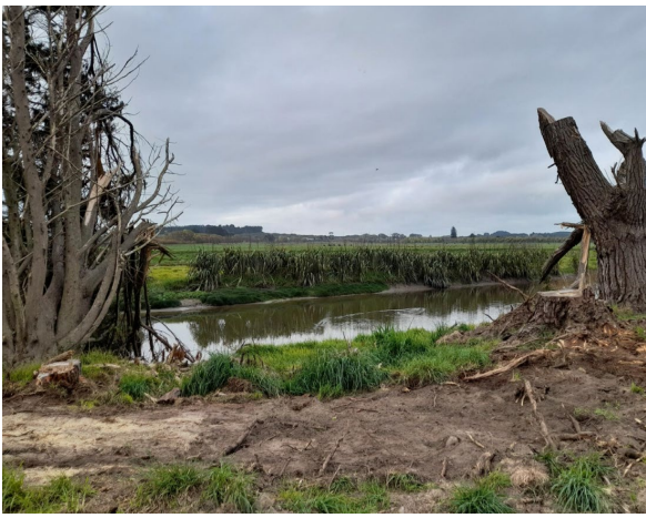
Surface preparation pre application of basecourse to Piriharakeke Walkway
