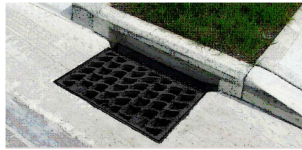
TYPICAL HYDRO STORM WATER GRATE AND FRAME WITH KERB BACK ENTRY (HYNDS TECHNICAL GUIDE SP2.5)
