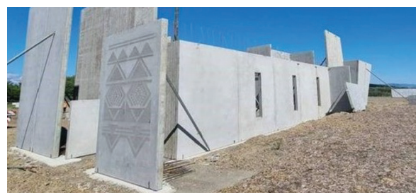
Panels and services are being installed at Waitārere Beach Surf Life Saving Community Facility.
