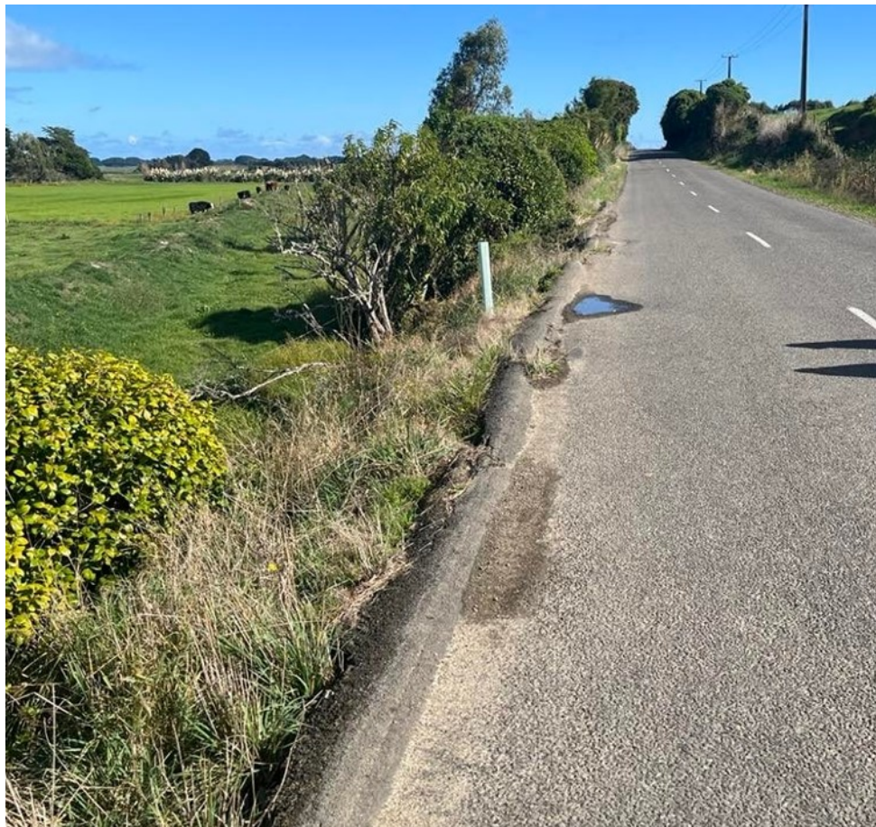
Figure 3 Koputaroa Road. An example of pavement deformation
