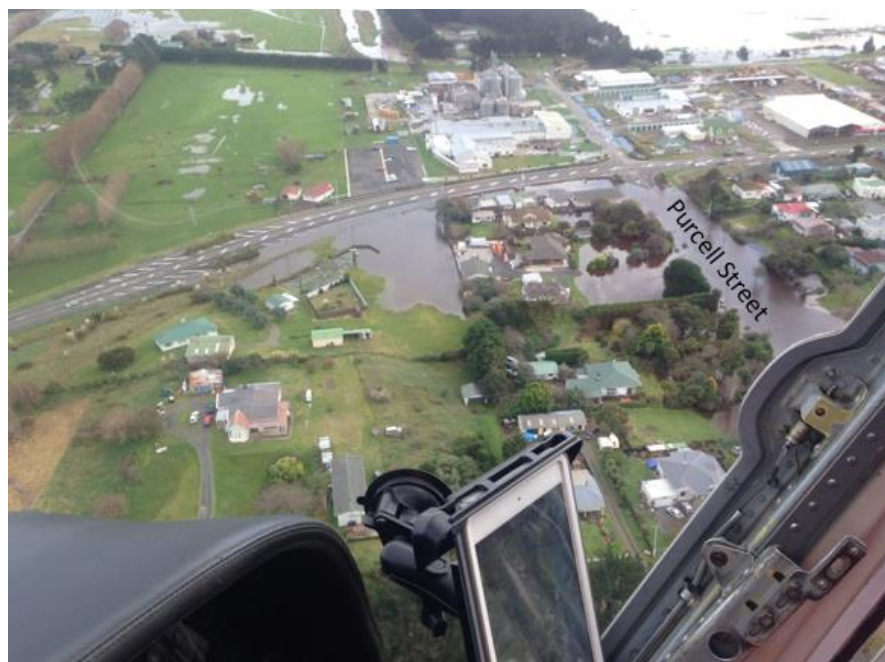
Photo 2: Purcell Street flooding – June 2015.
