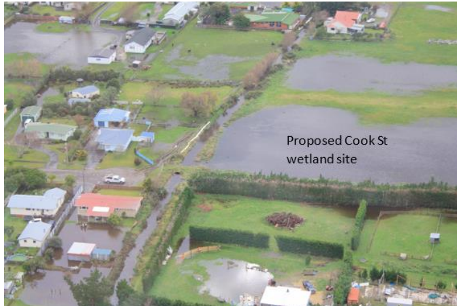
Photo 1: Wetland site (work package C & D) on true left bank of Kings Canal (inundated area) and sand bags to prevent overtopping on the true right bank – June 2015.
