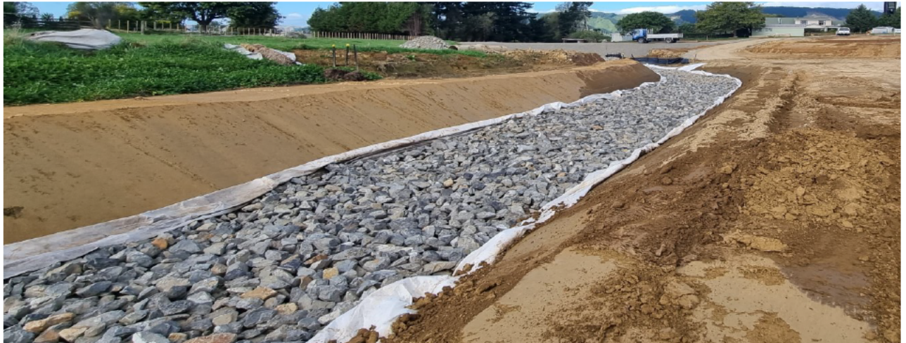
(High Flow bypass)
