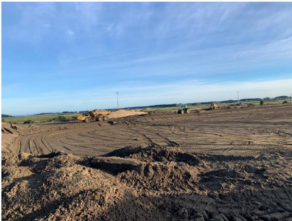
Figure 1 Construction of the western bund.
