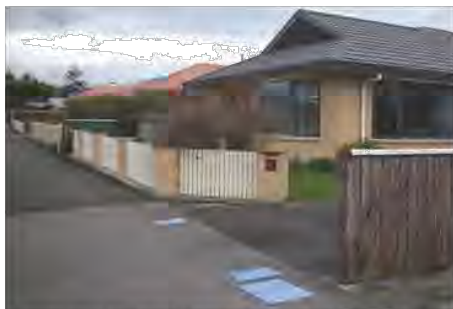
Uniform street frontage with a consistent setback along the street and low front fences
