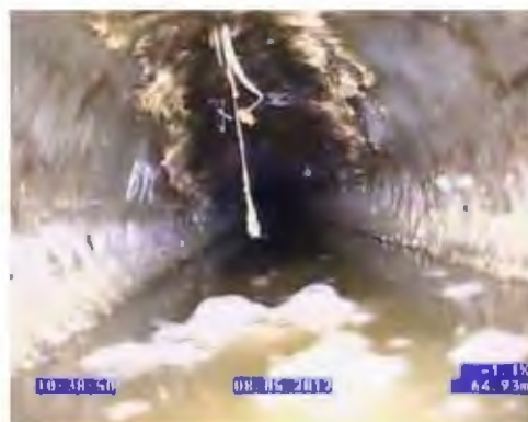
What lies beneath us - a blocked and broken wastewater main under Stafford Street, Shannon 2012
