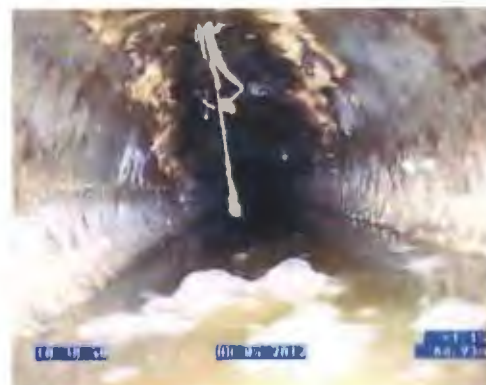
What lies beneath us - a blocked and broken wastewater main under Stafford Street, Shannon 2012
