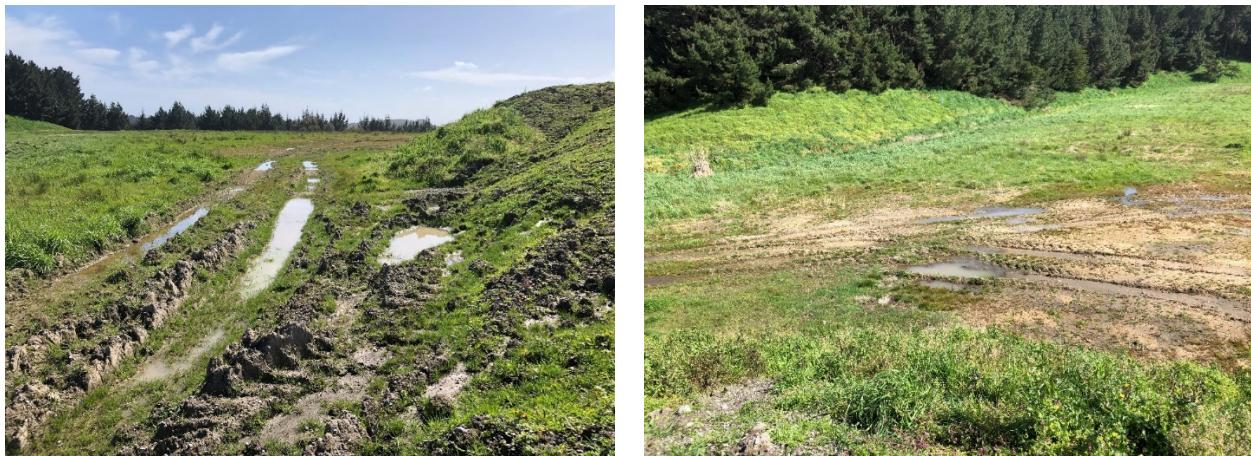
**Figure 11-2 Evidence of ponding on top of the old landfill caused by vehicle movements (20/09/21)**
