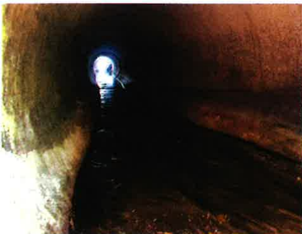
Photo 7 Looking through the culvert showing the pooling water, slowing the water velocity to allow fish to migrate through the culvert.
