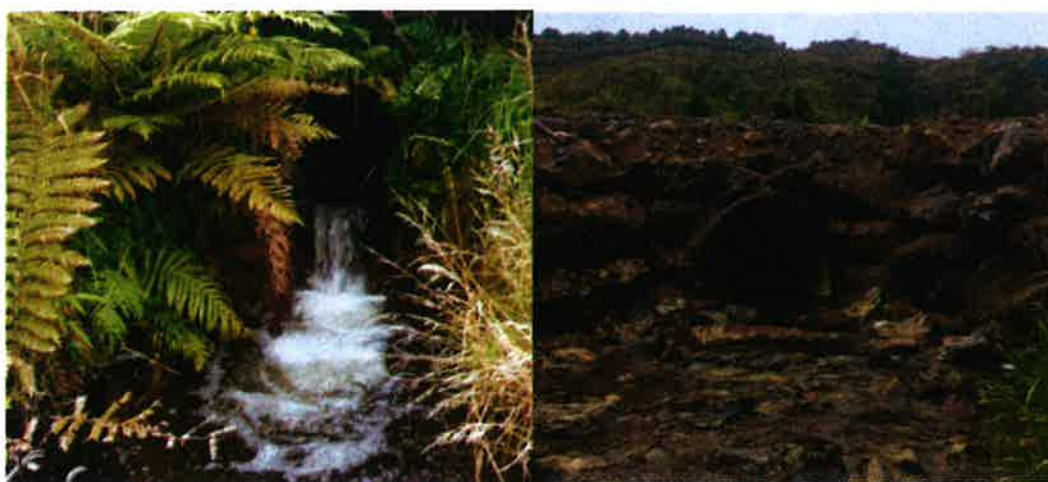
Photo 1 A perched culvert before and after replacement.
