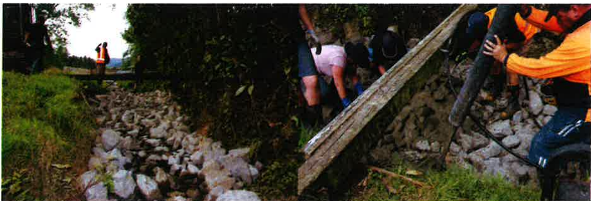
Photo 4 Final placement of rock for the correct gradient and start of concreting after water diversions are in place.
