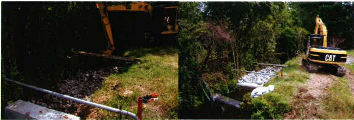
Photo 3: Installation of a slightly higher weir to flood the perch on the culvert and installation of rock work prior to concreting the rocks in place.
