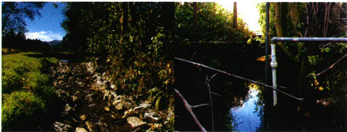
Photo 6 Left, weir after the concrete has dried and the water allowed to flow down the pass; right, raised water level flooding the culvert drop which will allow fish free access to upstream.
