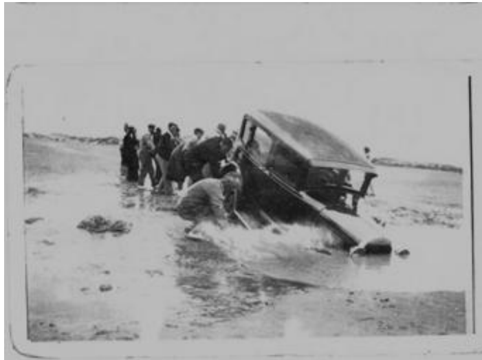
Figure 6 Liquefaction effects of an earthquake at Foxton Beach 1934 (Foxton Historical Society).
