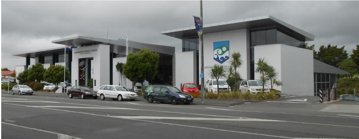
Fig.1: Horowhenua District Council Building
