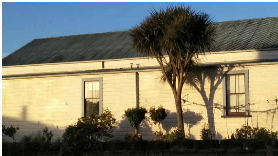
Side of the Tokomaru Community Hall that needs replacing.
