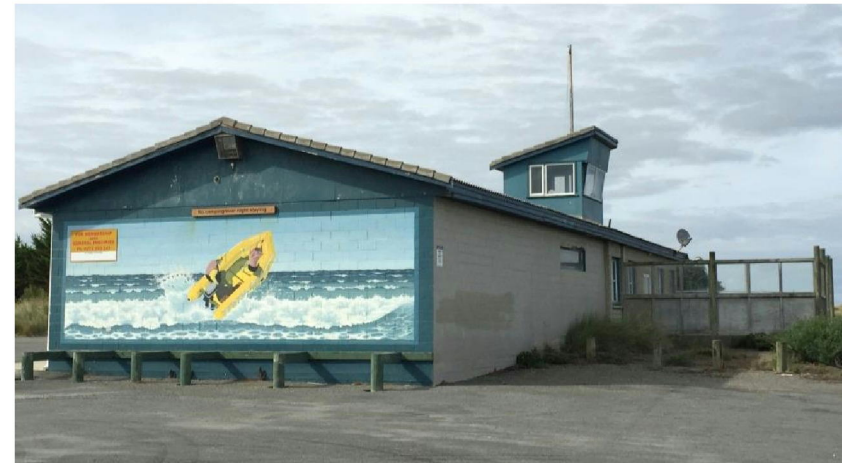
Image 11 Current Levin-Waitarere Beach Surf Lifesaving Club building
