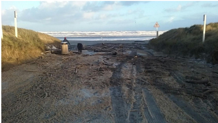
Image 8 Debris blocking the main beach access at Waitarere Beach following a storm (photo supplied by Recreational Services in July 2016)
