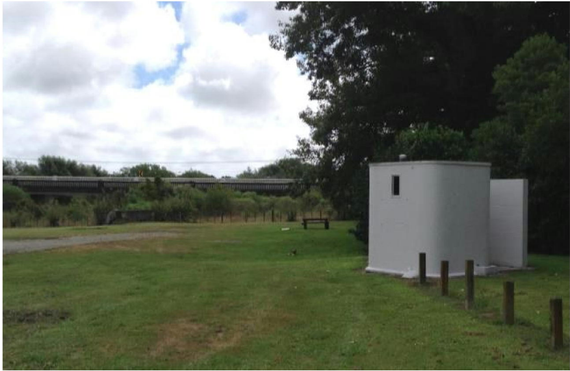
Image 12 Currently unused toilet block at Parikawau Reserve
