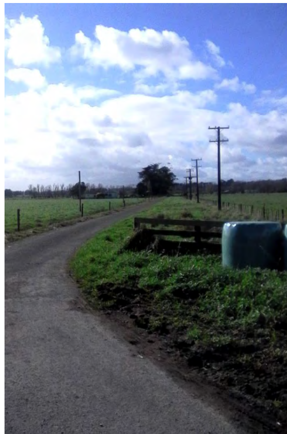
Looking North from Puketea St along Toitoi St this section is used as a roadway.
