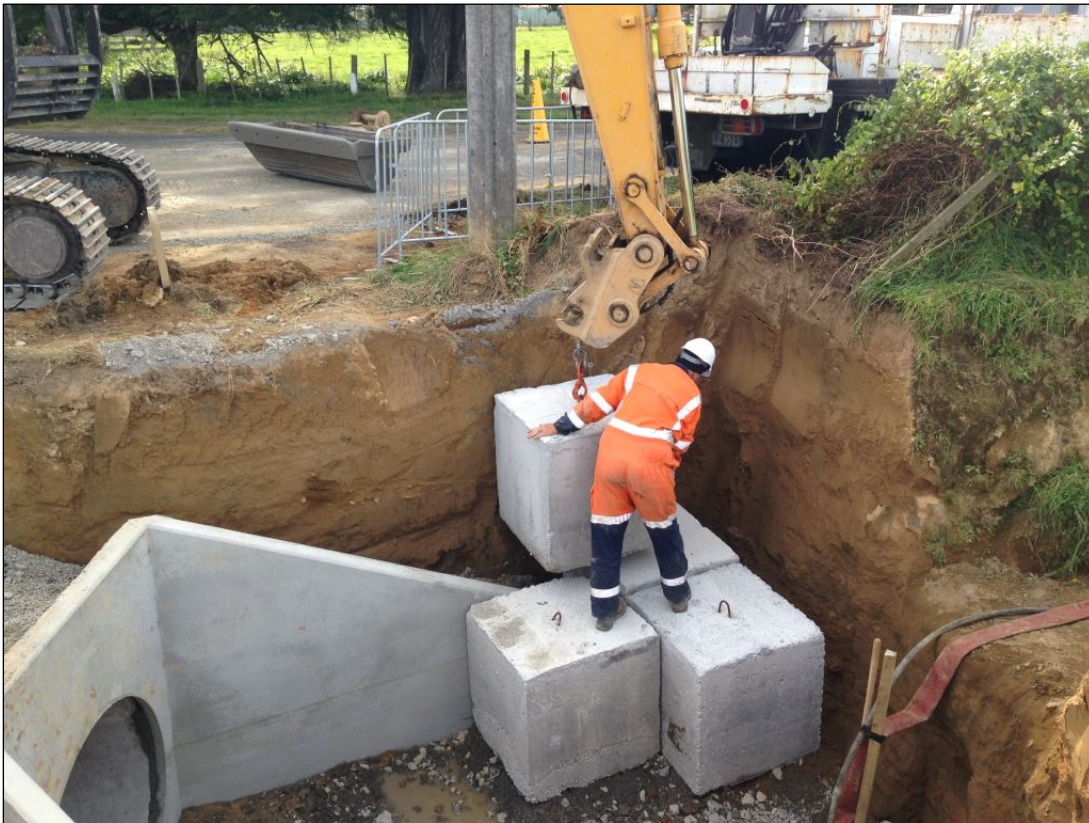
Temporary support of Electra pole at outlet structure. The pole may need to be moved. HDC will liaise with Electra to confirm this. (March 2017).
