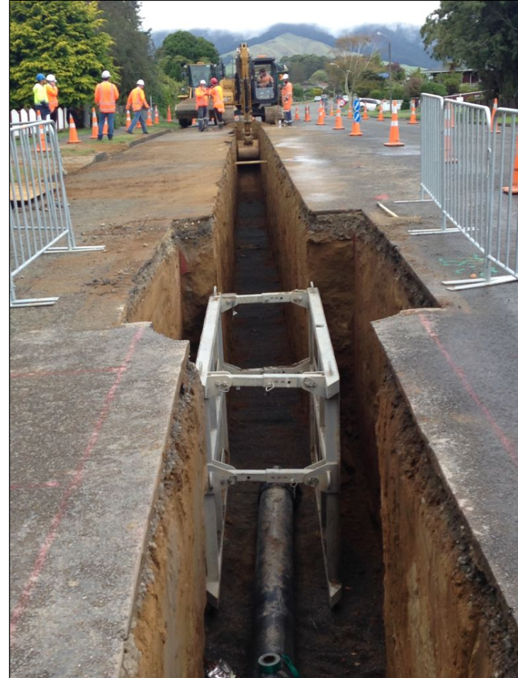
Excavation of trenches along Kennedy Drive – note trench shield to allow workers to safely weld pipe together (March 2017)
