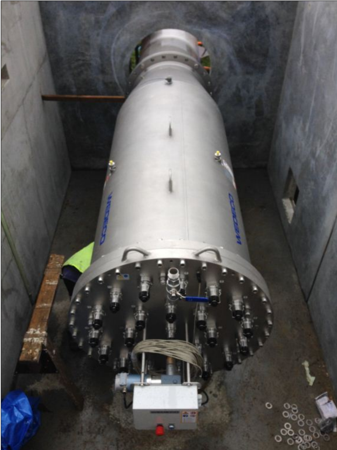
UV unit installed in building (Mar 2017)
