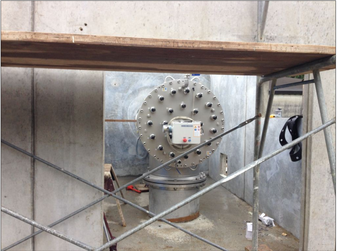
UV unit installed in building (Mar 2017)
