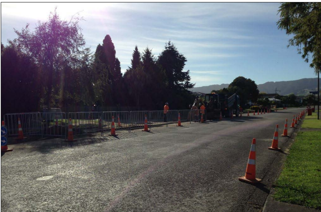
Kennedy Drive TMP in place and contractor excavating trench (March 2017).
