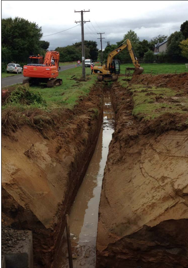
Deepening the drain downstream of pipe outlet – the new pipe invert level is approximately 1 m deeper than the old pipe invert level (March 2017).
