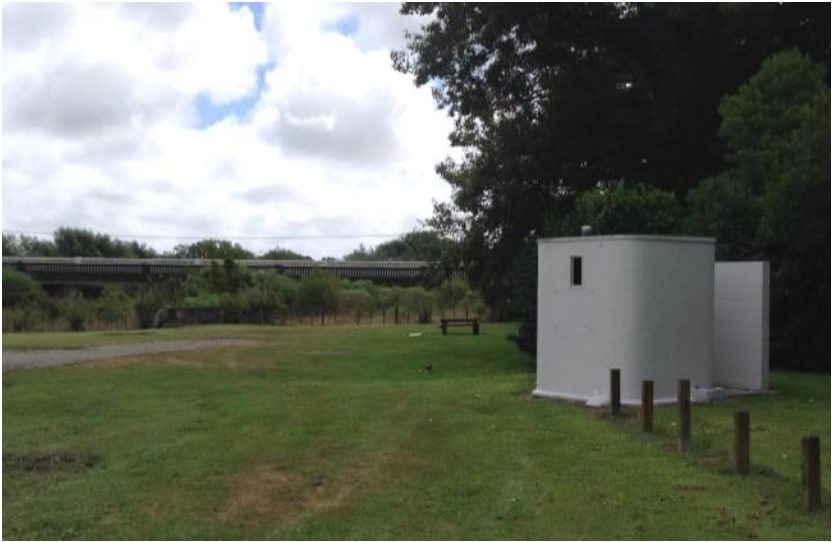
Image 12 Currently unused toilet block at Parikawau Reserve
