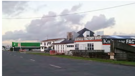
Photo 6: Cambridge Street South looking north towards wholesale trade supply (RD 1) and manufacturing industries. Buildings are a mix of styles, yet are similar in scale and alignment with the street.
