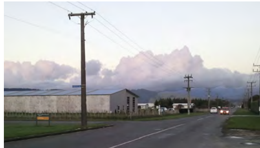
Photo 4: Looking west along Tararua Road, simple building form and structure.
