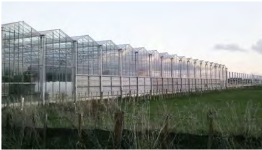
Photo 3: Looking south-west along Tararua Road towards adjacent Rural Zone. The form and scale of the glasshouses provides distinctive character of the locality and their functional use.
