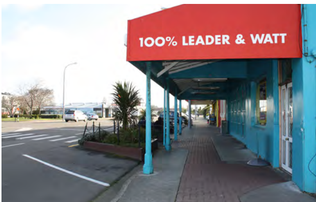
Verandah posts on Main Street, Foxton
