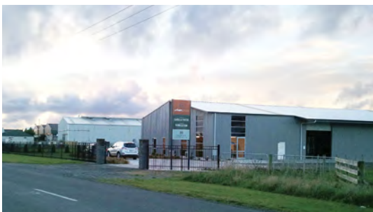
Photo 1: Looking west along Tararua Road. Established industrial activity. Rural industrial character. Single storey workshop/warehouse, simple pitched roof.
