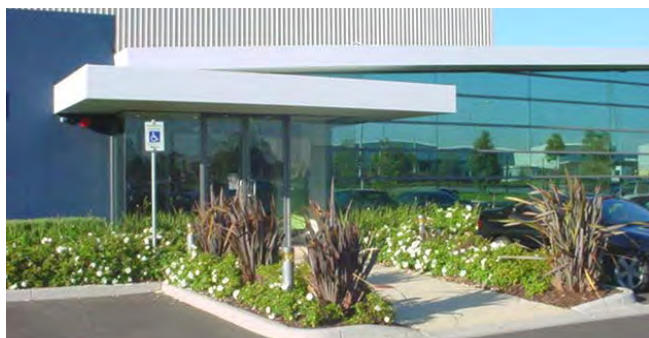
1. Primary (visitor) access and building frontage
