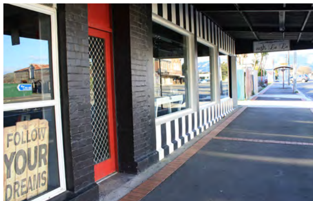
Glazing on Ballance Street, Shannon
