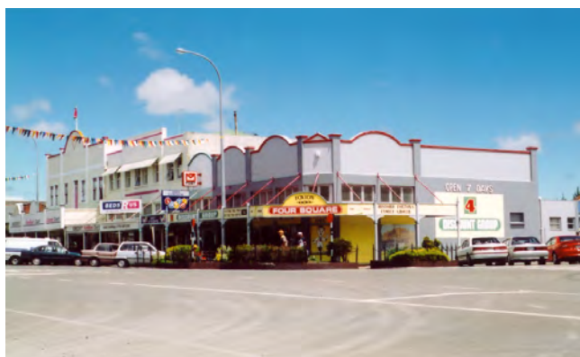
Figure 5: Building on corner of Main Street and Clyde Street, Foxton
