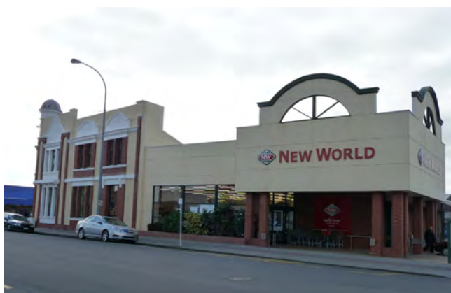
Retention of Whytes Hotel facade and new supermarket, Main Street, Foxton
