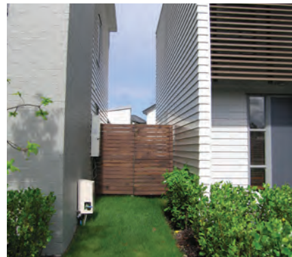
Utility areas separate from parking & screened from street
