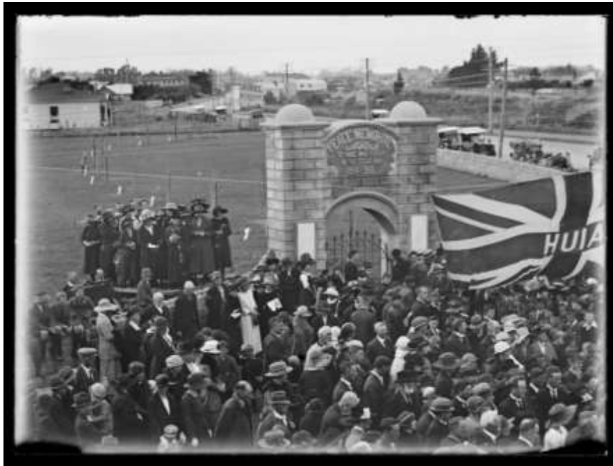
Figure 17 A scene from the unveiling the Weraroa Peace Memorial on 11 th April 1923. The line of young trees in the background will have been the pioneer trees. This photo shows the proximity of the memorial to Oxford Street in the background. The flag being used is the Ngati Huia flag 'Huia', which was also used for the 1903 'Welcome Home' parade following the South African War, 1 thus the use of this particular flag for the memorial unveiling was symbolic in itself. This flag was also flying in a photo of the Kikopiri meeting house, Muhunua West Road, Levin, in around 1910. 1 (Photo: Leslie Adkin. Gift of G. L. Adkin family estate, 1964. Te Papa [B.022273]: http://collections.tepapa.govt.nz/object/109681 )
