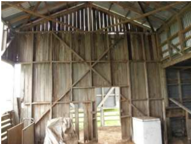
Figure 61 The interior of the old shed, showing an original wall. It is not clear if it was built as a hayshed or as a mill building, but evidently ventilation was a necessity for it - Whitaunui site, 11 th May 2016
