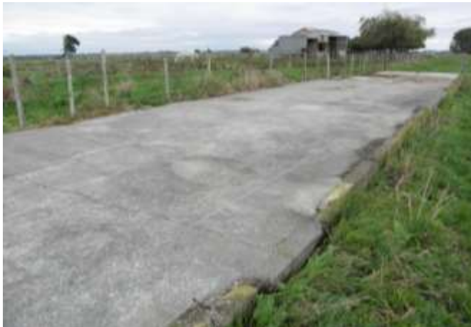
Figure 58 Old and new concretework that now forms a cowshed race. The old wall includes protruding steel reinforcing. The original building possible relates to the flaxmill. The old shed detailed below, is in the distance - Whitaunui site, 11 th May 2016
