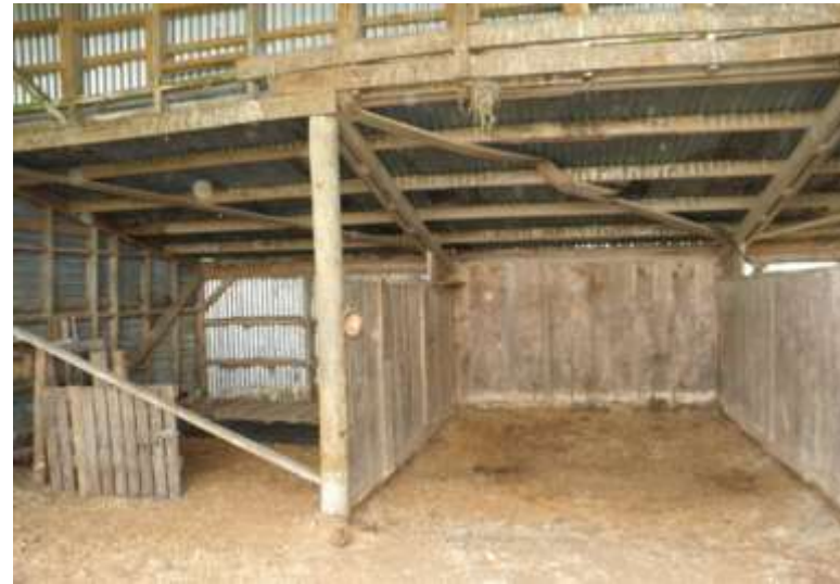
Figure 62 One of the three bays inside the old shed. This is the only one (now) lined with timber, much like a loose box might be, but it is not possible to know when the lining was installed - Whitaunui site, 11 th May 2016
