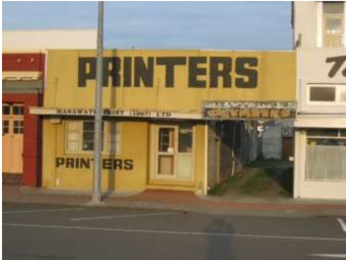
Figure 31 The building with its tired and somewhat underwhelming stucco façade, before work began in 2015. Former owner, John Read, began working there in 1959/60 and has no recollection of the building having this façade added, and it is believed to date to the 1940s. (Photo: Jim & Sarah Harper)
