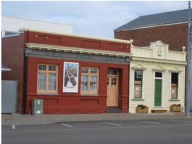
Figure 33 The completed exterior, alongside the former Foxton Racing Club building, in 2016. Both buildings belong to the Harpers (Photo: Jim & Sarah Harper)
