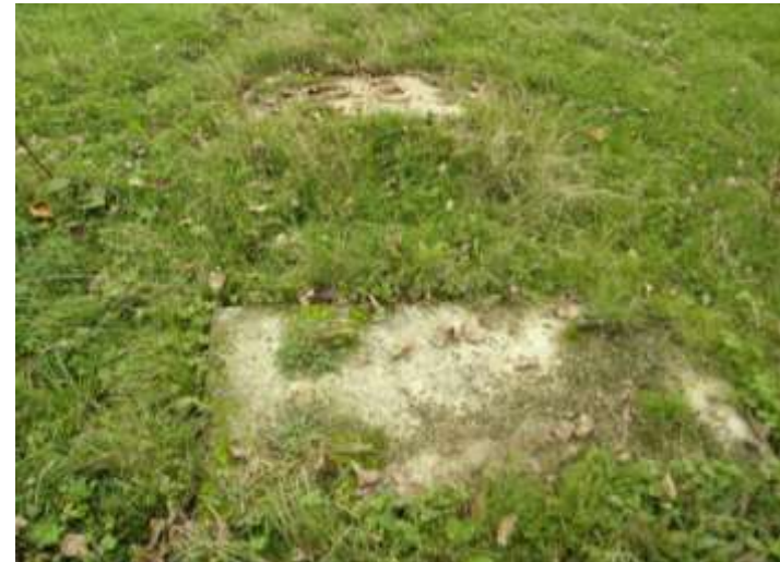
Figure 57 Part of the flying fox system. Both of these concrete blocks have four steel rods protruding from them suggesting that they once carried an engine and/or winch associated with the flying fox. A steam winch was employed at the flaxmill for this purpose - Whitaunui site, 11 th May 2016
