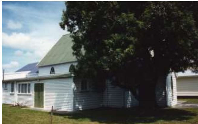
Figure 12 This photo shows the original portion of the building on 3 rd January 1996, along with some of the alterations that have occurred since 1972, in the course of re-purposing the building. (Photo: Val Burr)
