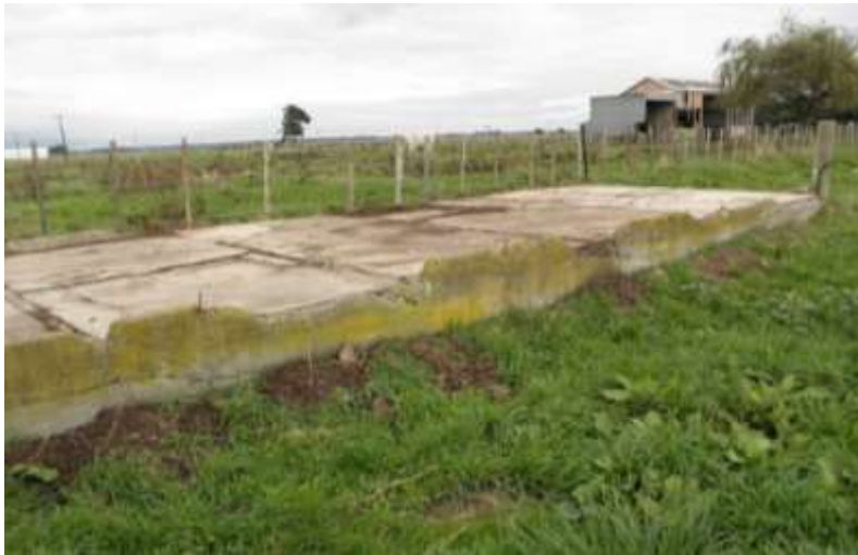
Figure 56 Old concrete foundations with reinforcing steel protruding from them, now used as a cowshed race, alongside the present cowshed. It is possible that they are part of a previous cowshed or something re-used from the flaxmill days. Whitaunui site, 11 th May 2016.
