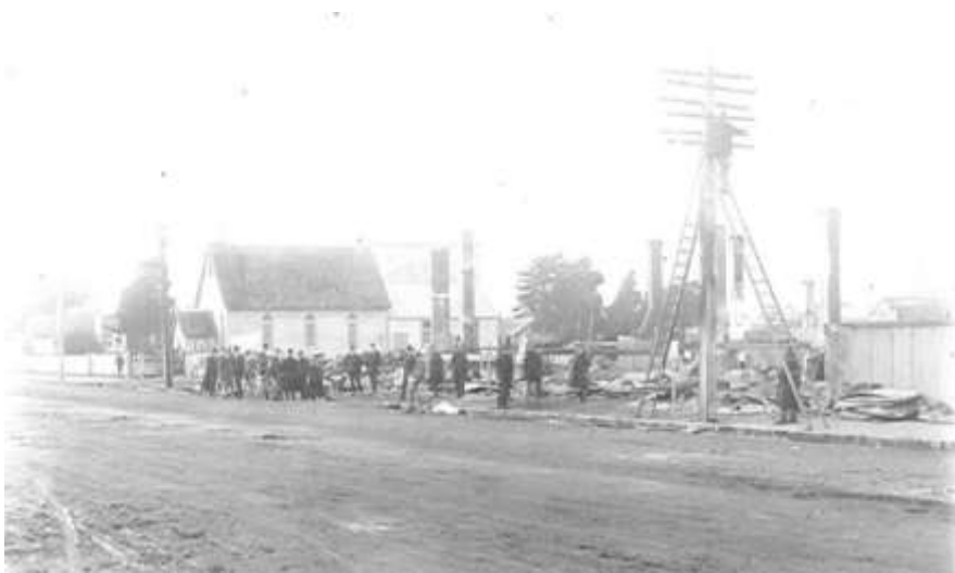
Figure 8 This scene is the eastern side of Main Street, Foxton, probably just hours after the early-morning fire of 23 rd July 1912. Foxton Presbyterian Church is in the background, and notes on the reverse of the original photo state: “Mark on church roof below belfry is one of two places where roof caught fire. The fire had to be stopped at this point.” Note also the extension on the back of the building. (Source: Photo ID: f1999.0220, Foxton Historical Society: http://horowhenua.kete.net.nz/site/images/show/5741-main-street-foxtton-after-the-july-1912-fire )
