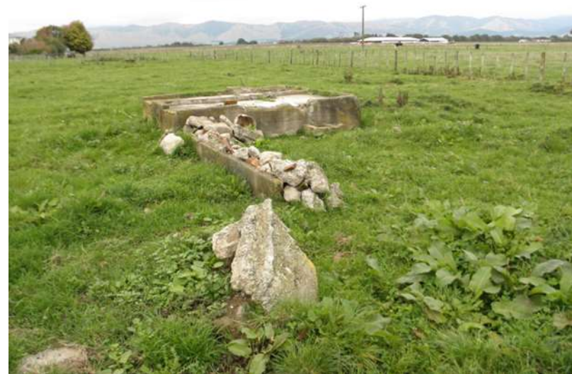
Figure 49 Foundations of an old toilet and shower (?) block – Whitaunui site, 11 May 2016. The detention camp’s accommodation ‘paddock’ is in the background beyond the foundations.
