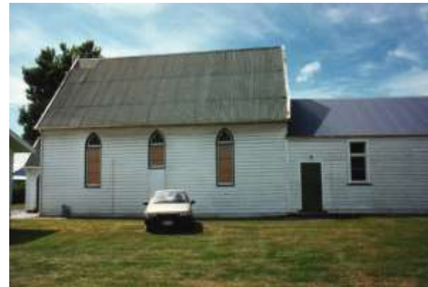
Figure 11 This photo shows the original portion of the building on 3 rd January 1996. This extension was also present by the time of the 1912 fire, pictured above. Note that the window that has been altered to accommodate a fire escape door for the Little Theatre. The patch of different-looking roofing iron shows the former location of the church's belfry. (Photo: Val Burr)
