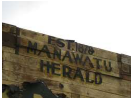
Figure 32 The old Manawatu Herald sign rediscovered beneath the stucco in 2015 – some of which is still visible at the bottom of this photo. This sign differs significantly from the two sign boards shown in the old photos of the building. (Photo: Jim & Sarah Harper)
