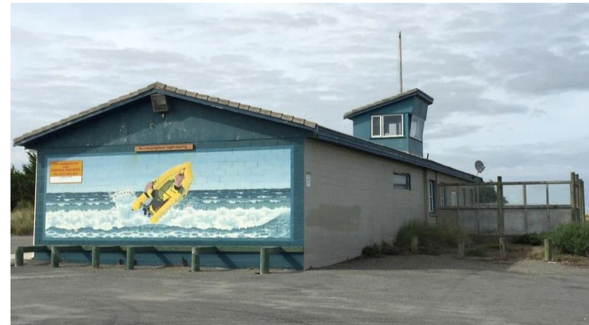
Image 11 Current Levin-Waitarere Beach Surf Lifesaving Club building
