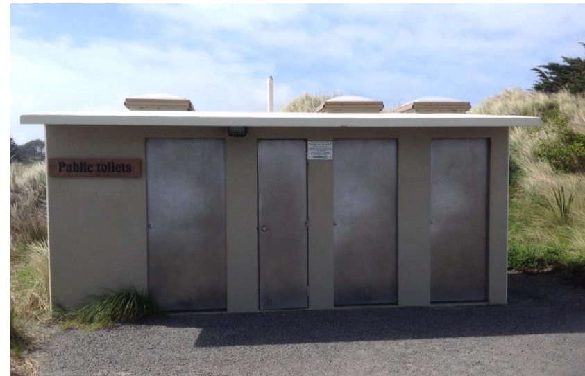
Image 13 Public toilets in the car park at Waitare Beach
