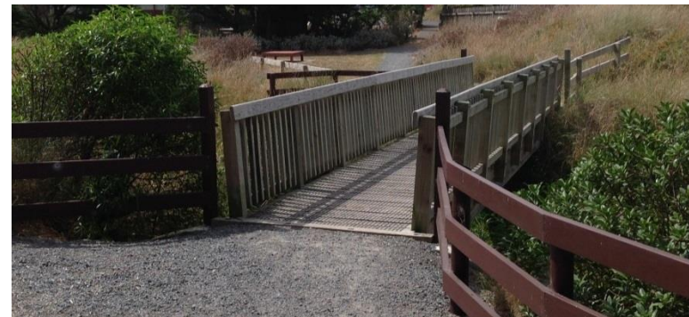
Image 18 Pedestrian bridge which crosses Wairarawa Stream near Somerset Grove
