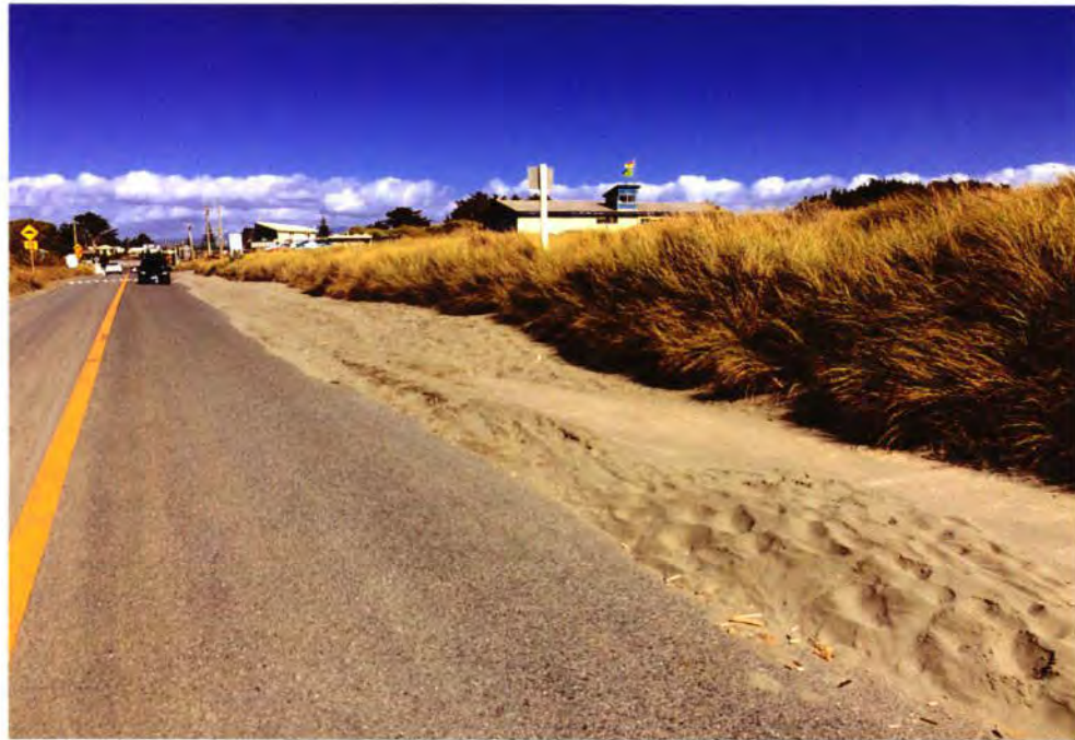
Footpath and verge build up 2017
